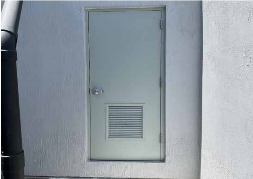
Door - Roof Storage
