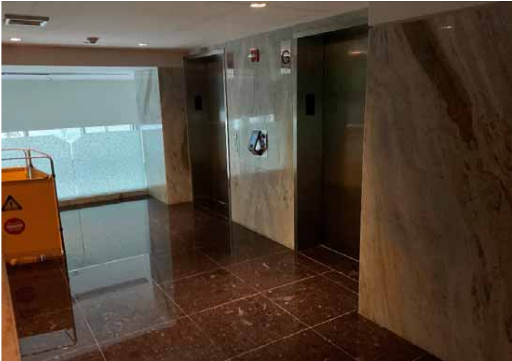
Elevator Lobby - Mezzanine Level
