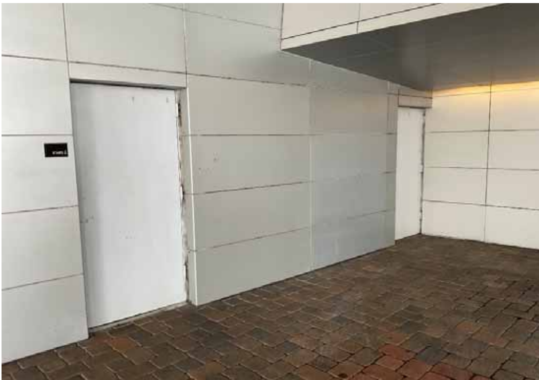
Doors - Garage Access
