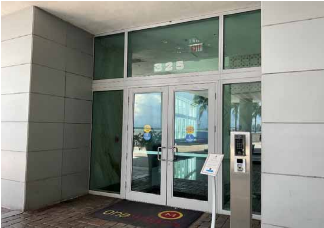
Windows & Doors - Lobby
