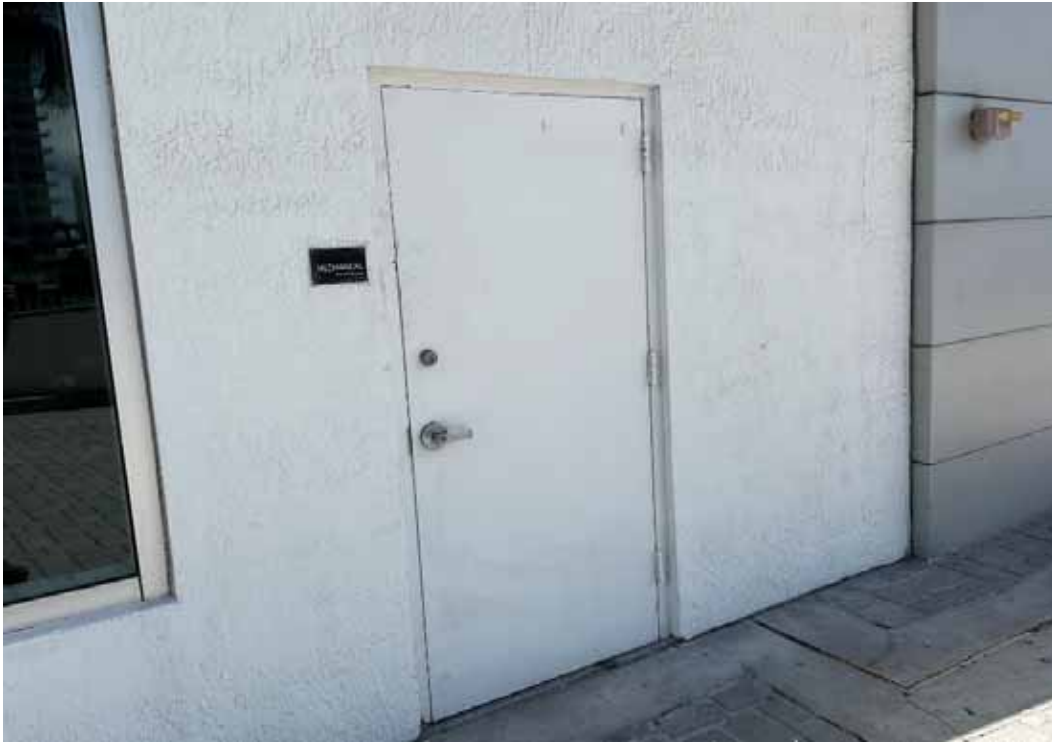
Door - Mechanical Room
