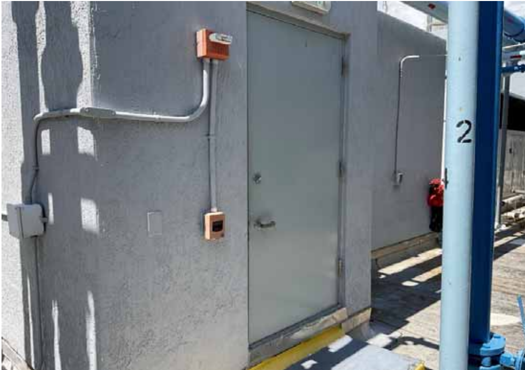
Door - Roof Access
