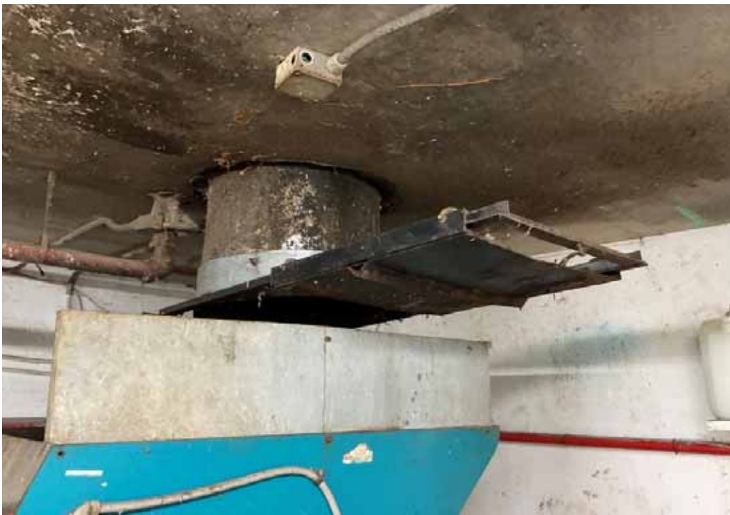
Trash Chute Guillotine
