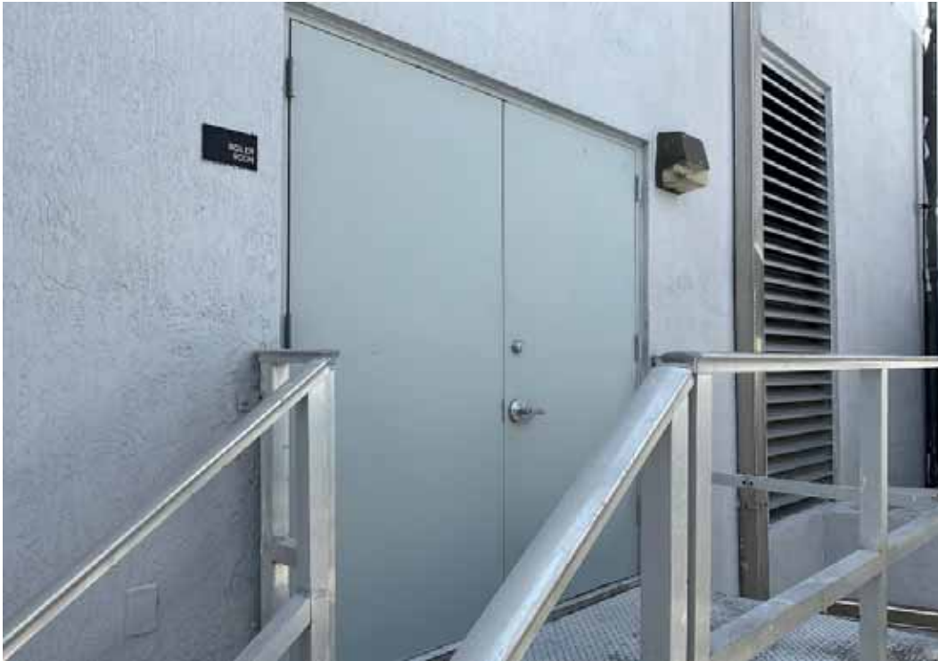
Doors - Boiler Room
