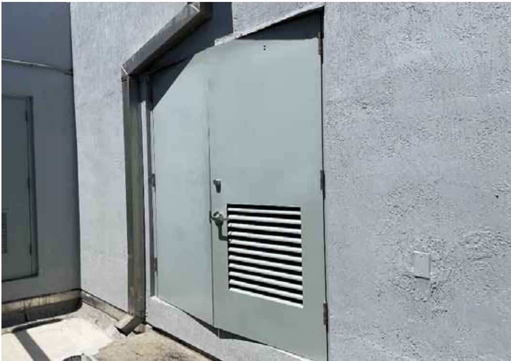
Doors - Roof Electrical Room
