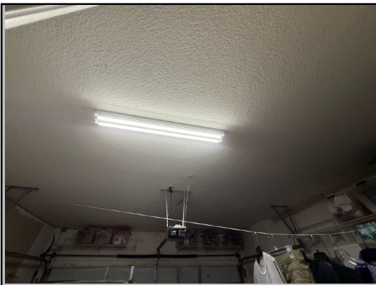
No signs of active leaks
