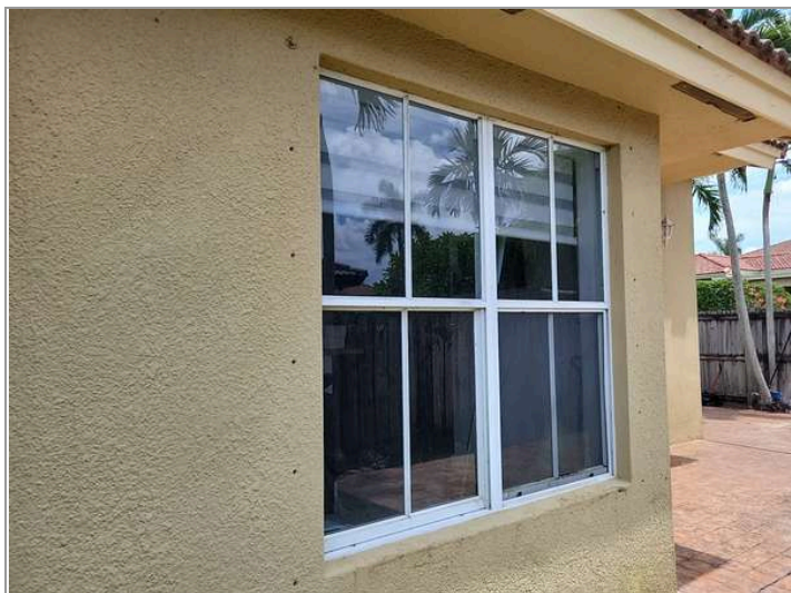
Rear windows shutter protected
