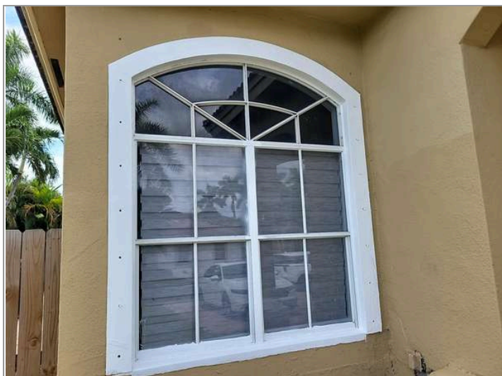
Front windows shutter protected
