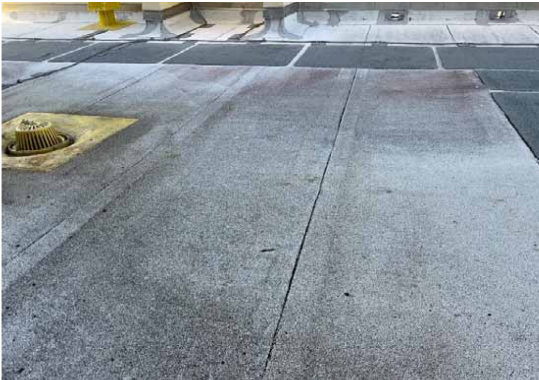
South Tower Roof
