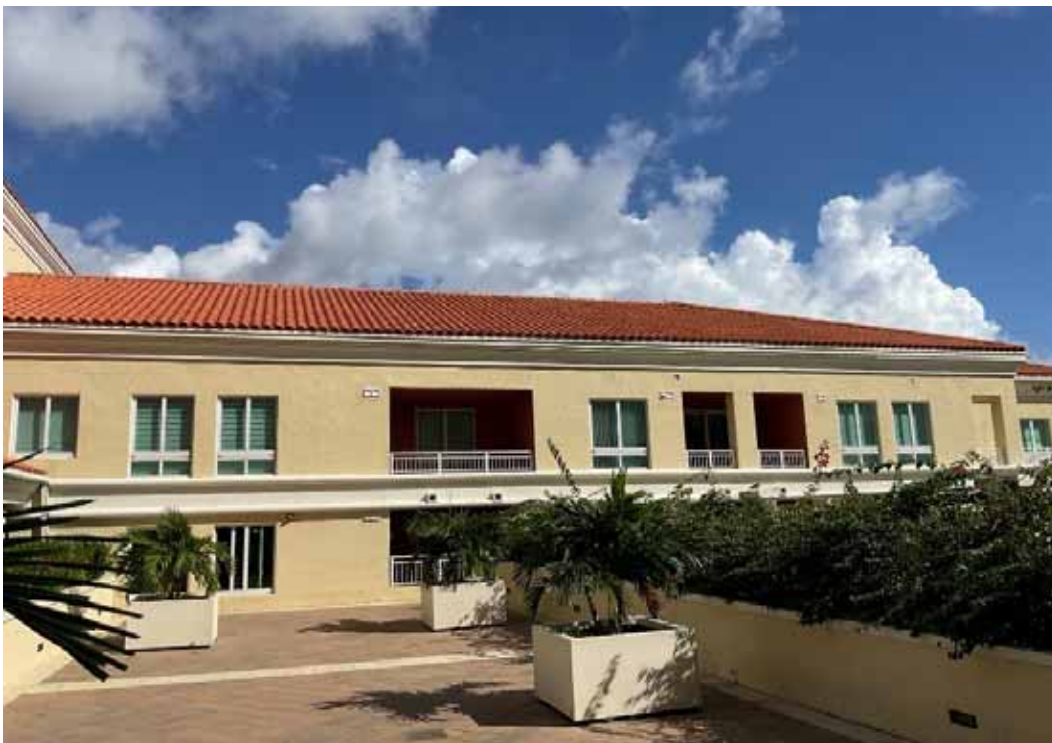
North Tower Roof
