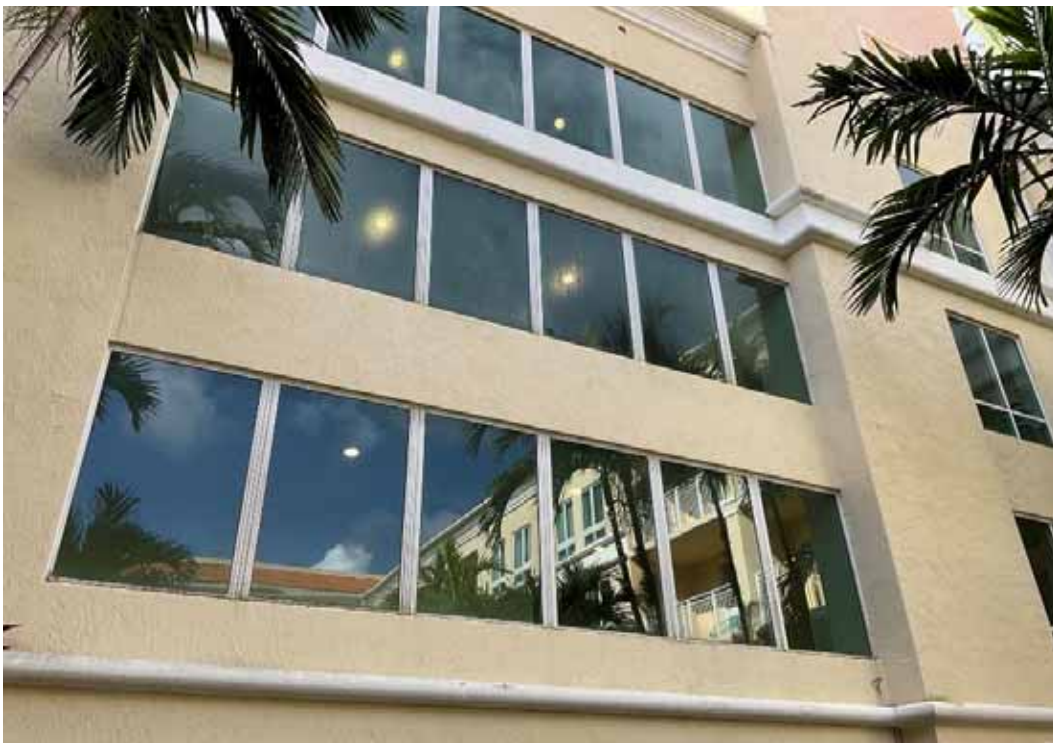
Windows - North Tower Hallways
