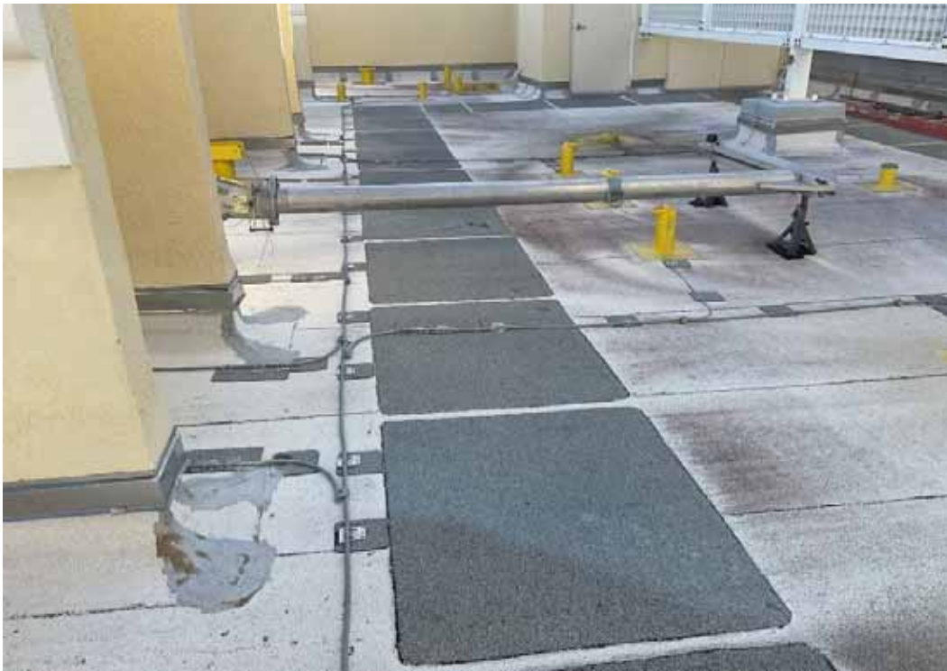
South Tower Roof
