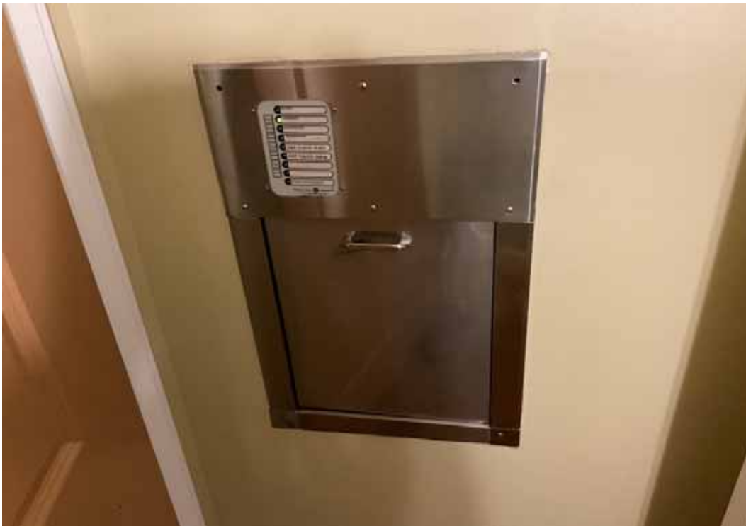
Trash Chute Door - South Tower
