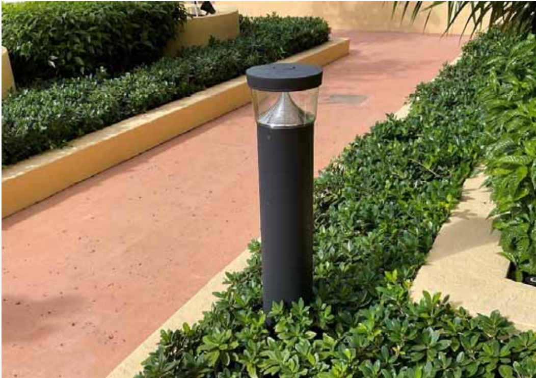
Light Bollard - Recreation Deck
