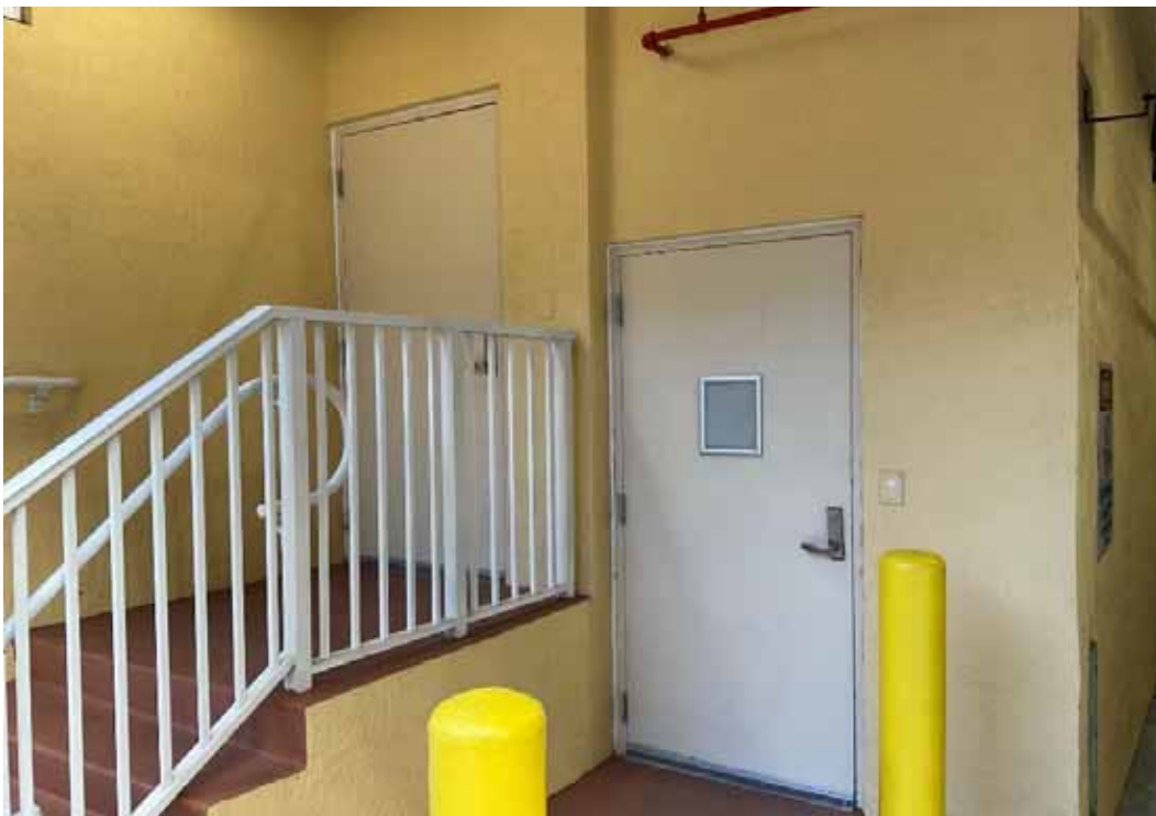
Doors - South Tower Service Areas
