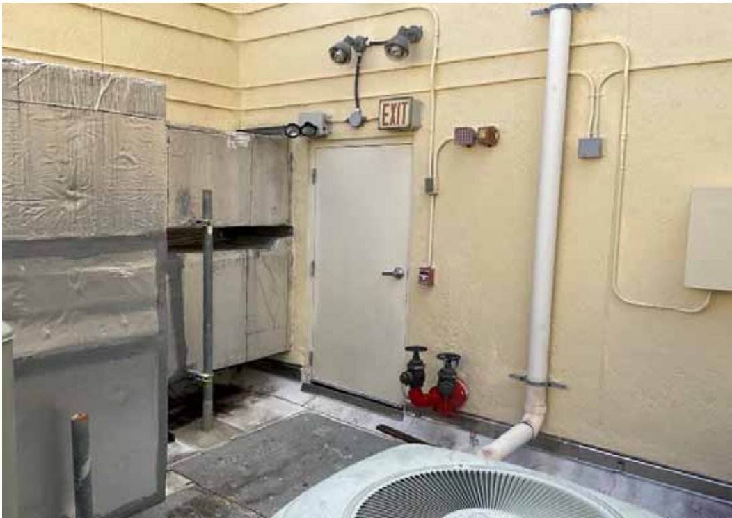
Door - North Tower Roof Access
