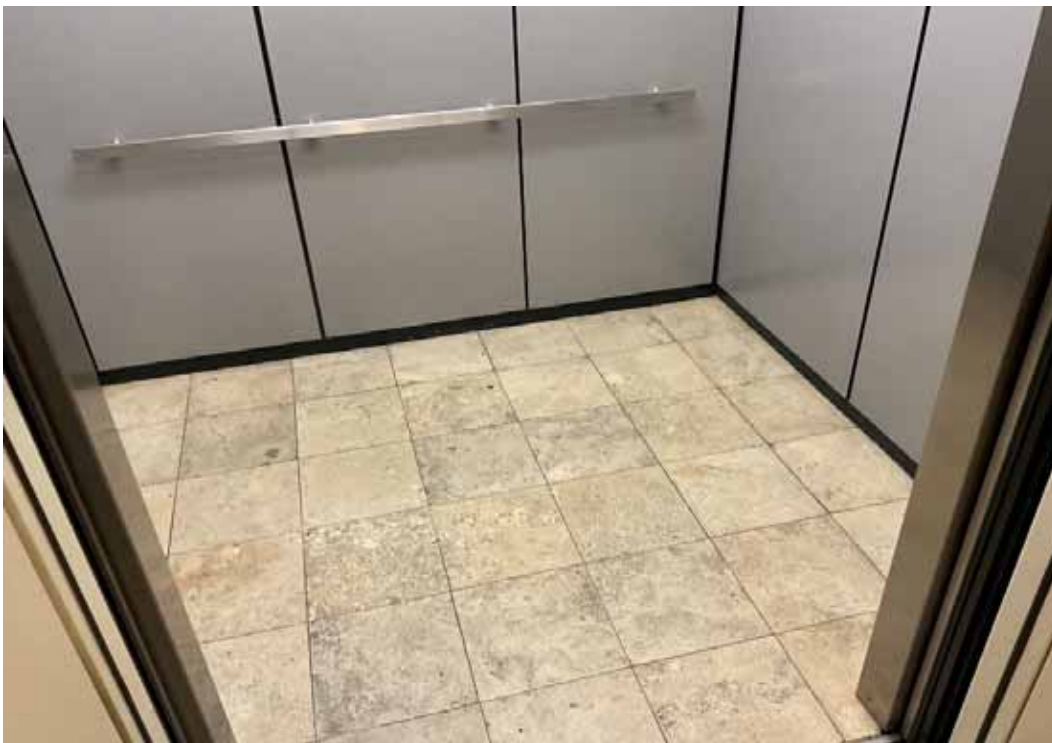
Elevator Cab Interior - Garage
