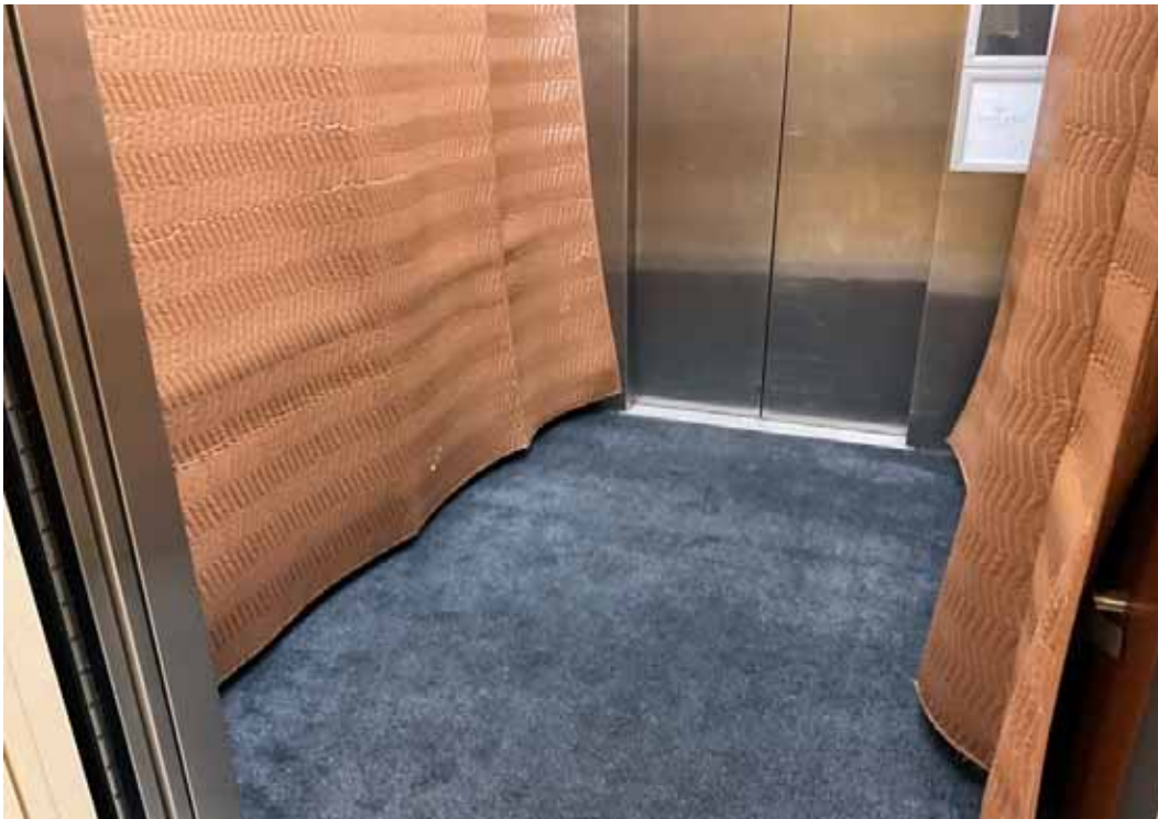
Elevator Cab Interior, Service - S Tower
