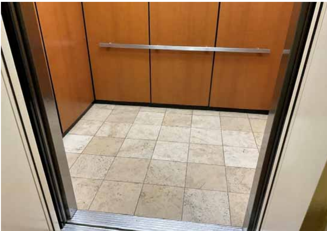
Elevator Cab Interior, Passenger - S Tower
