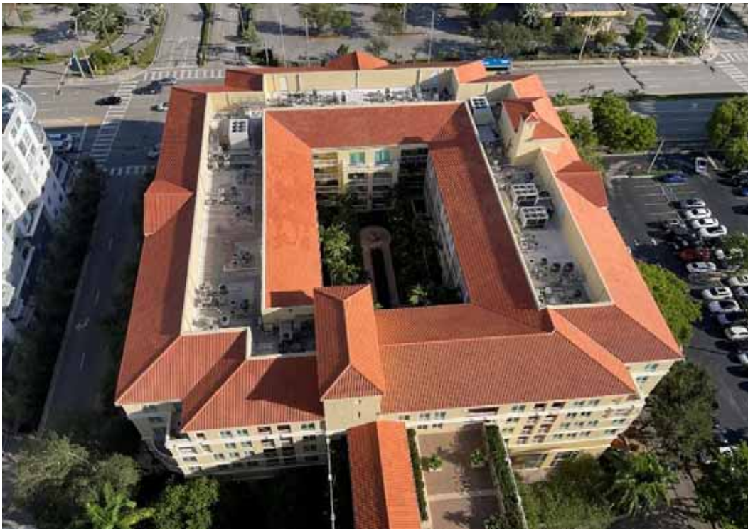
North Tower Roof
