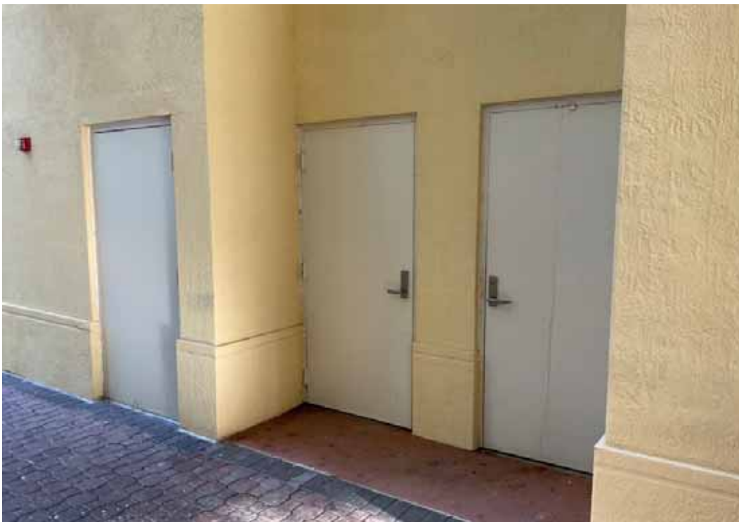
Doors - North Tower Service Areas
