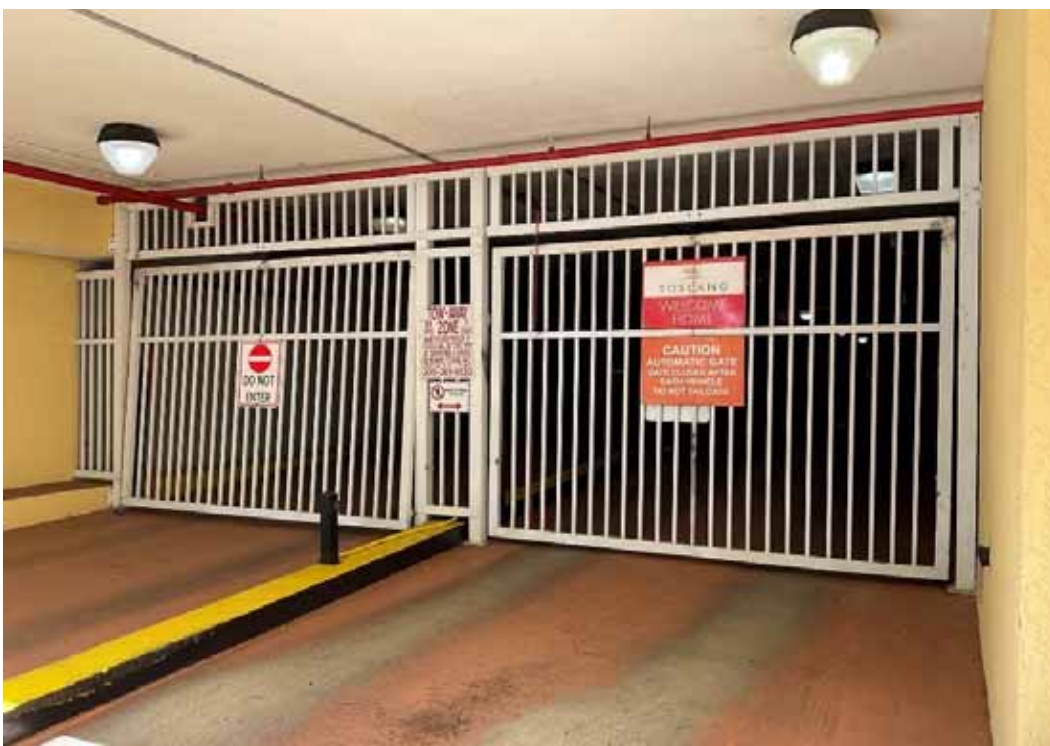
Garage Gates - Level 1
