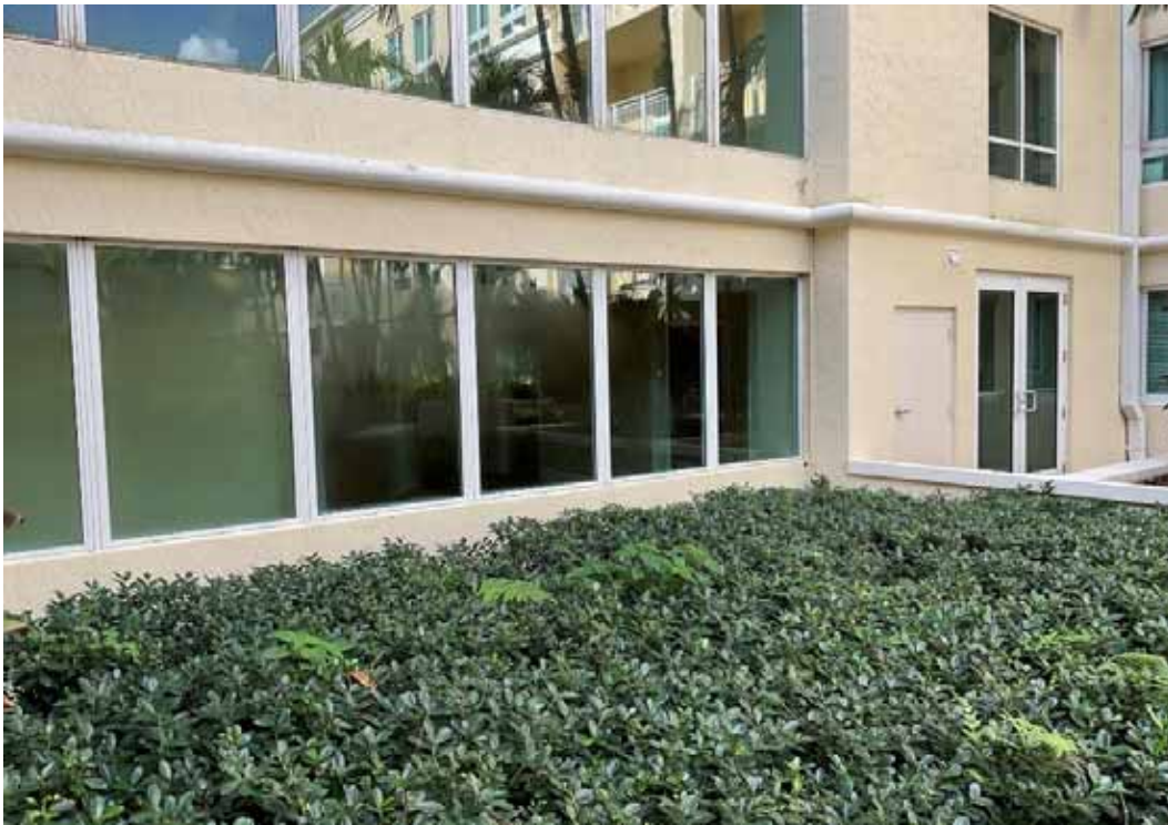
Windows & Doors - North Tower Hallways
