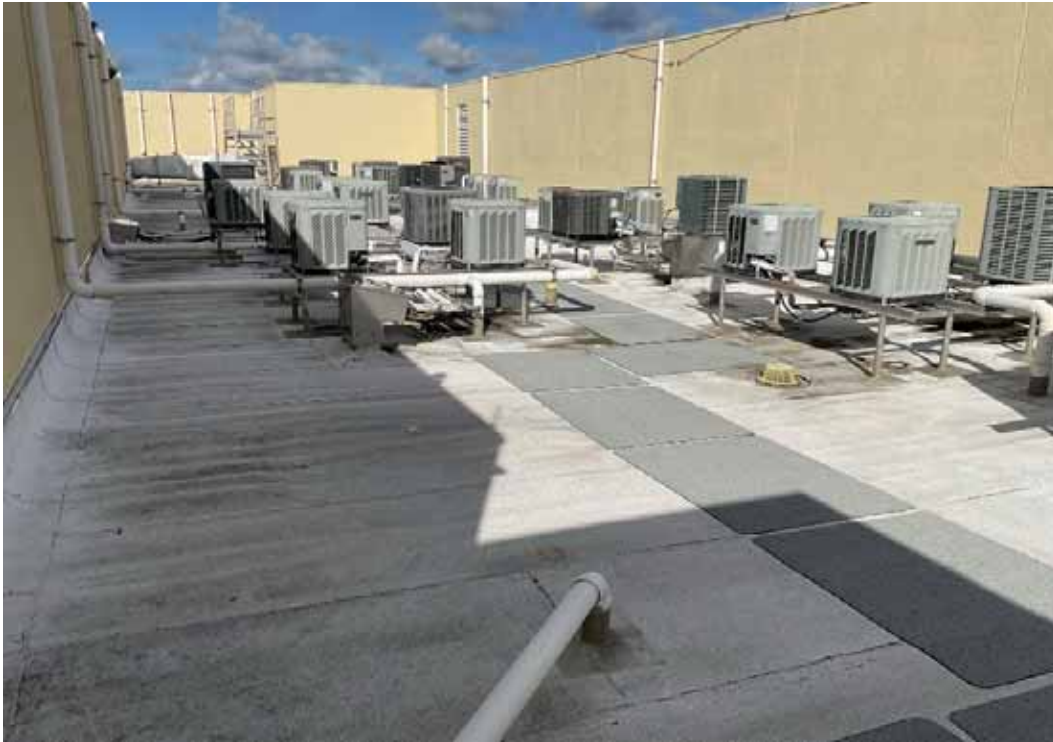
North Tower Roof
