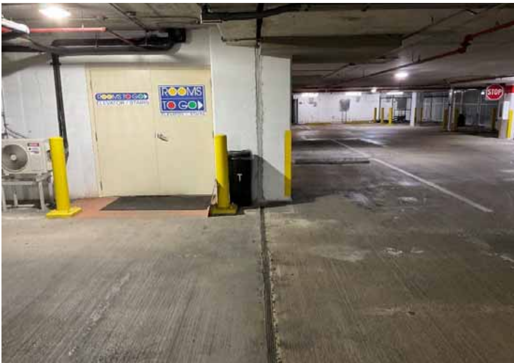
Garage Expansion Joint
