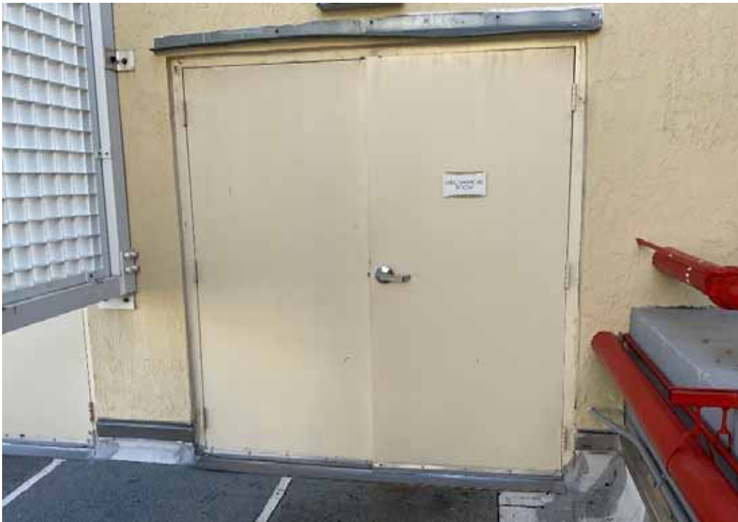
Doors - South Tower Roof Mechanical Room
