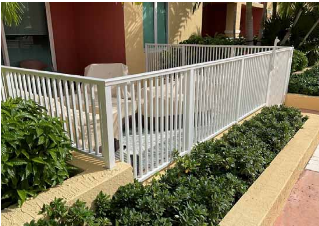
Balcony Railings - South Tower
