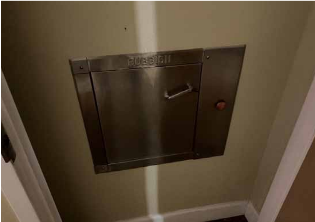
Trash Chute Door - North Tower
