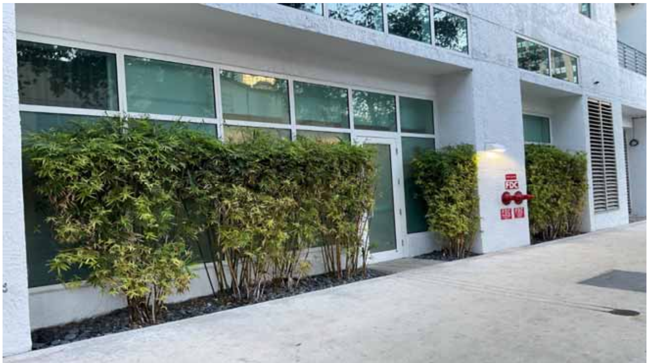
Windows & Doors - Main Lobby West
