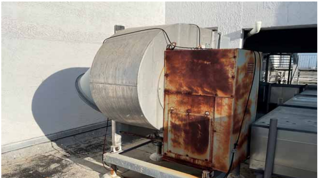
Stairwell Pressurization Fan - Hallways East
