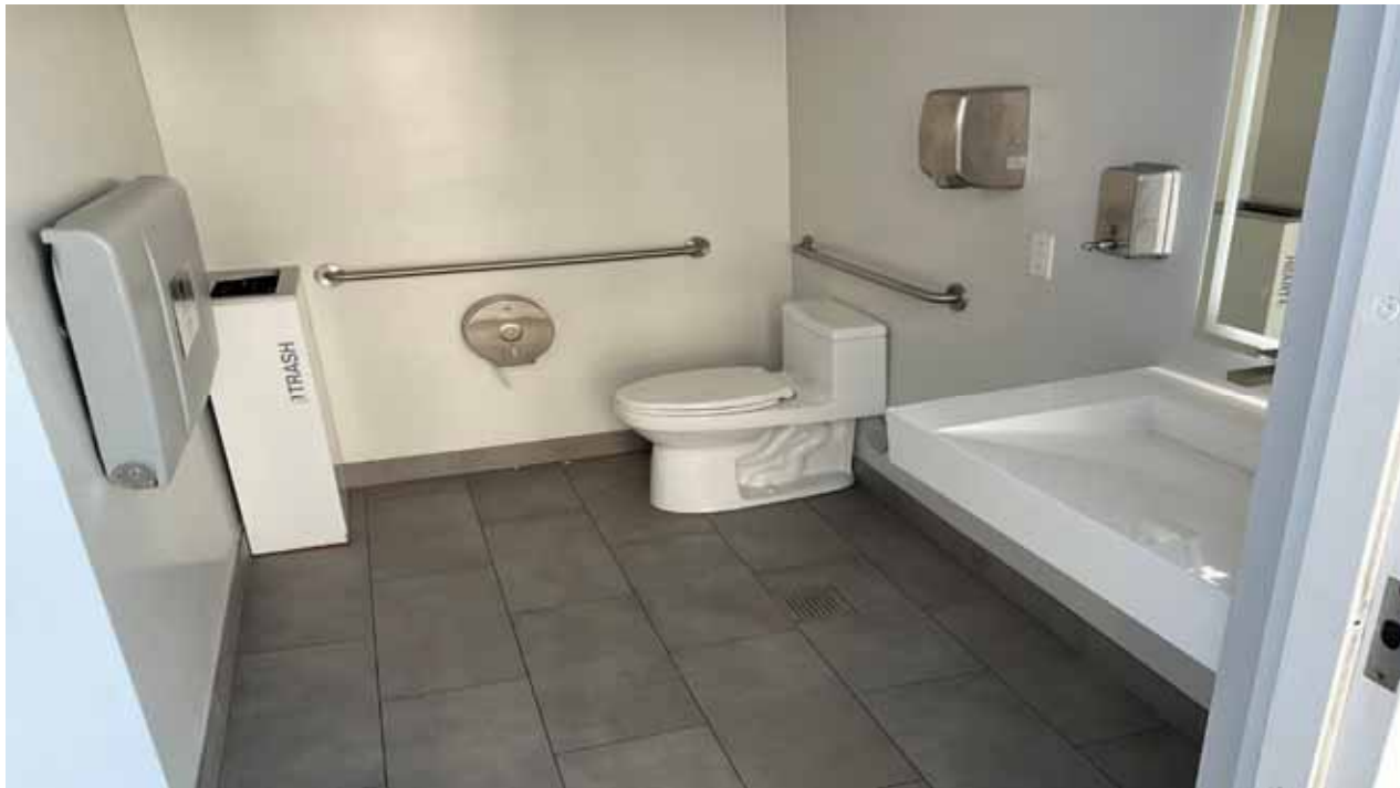
Pool Restroom, Unisex - Rooftop
