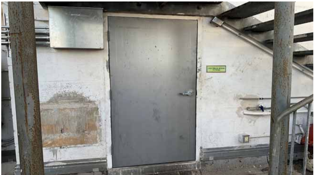
Door, Roof Electrical Room - West
