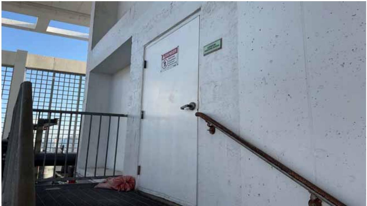
Door - Elevator Equipment Room, West
