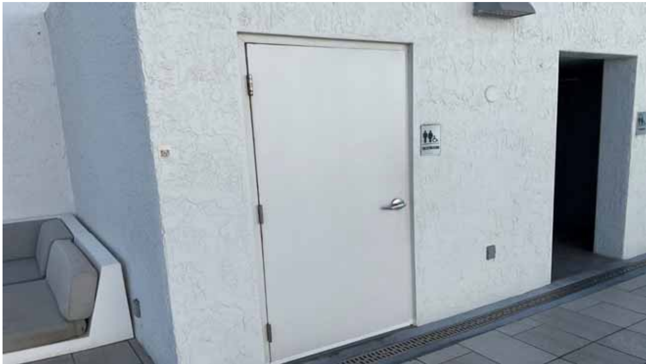
Door - Pool Restroom, Rooftop
