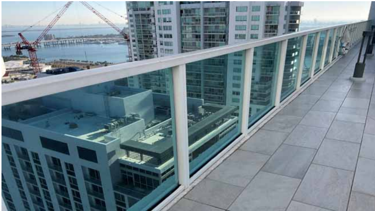
Pool Deck Railing
