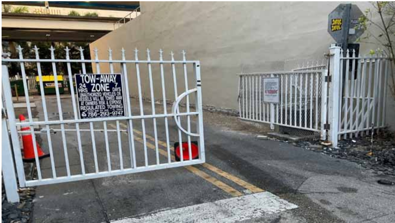
Gates - Receiving Area
