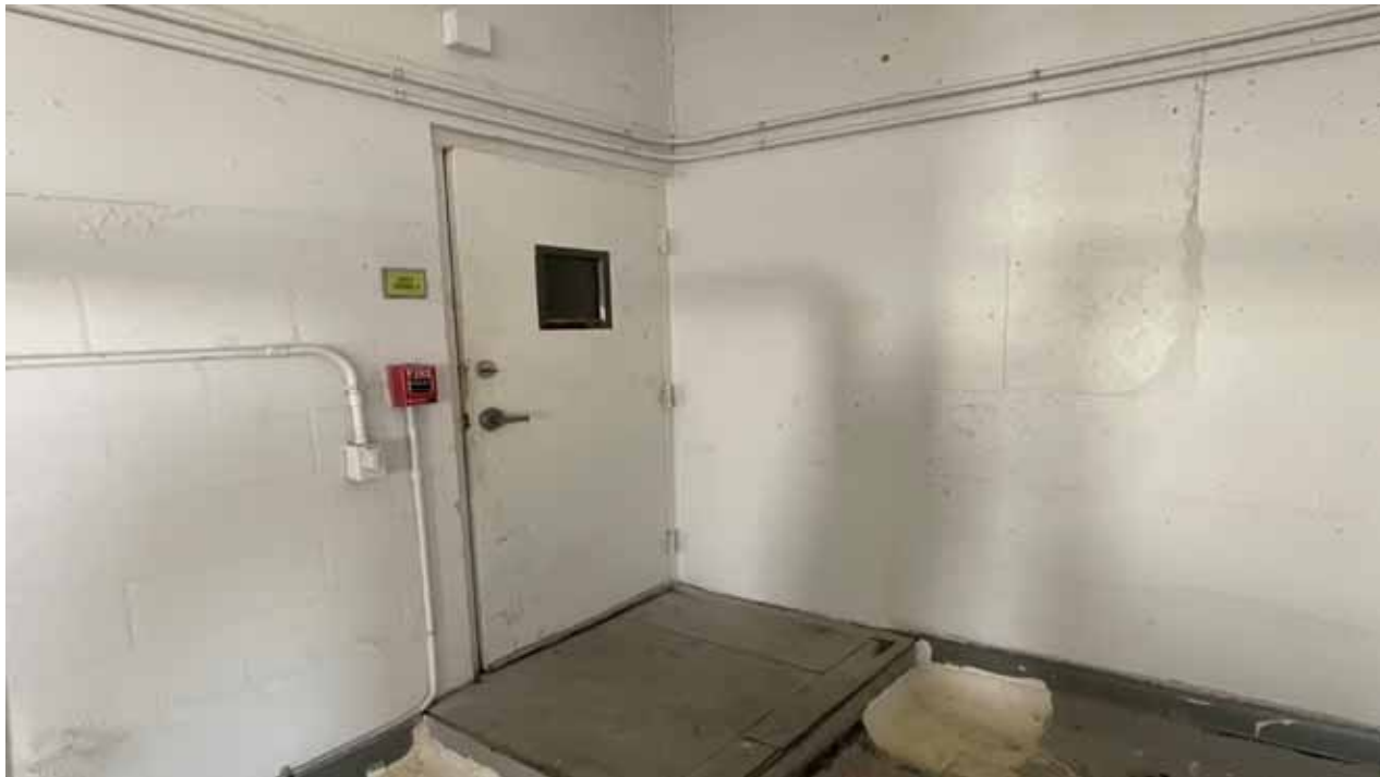
Door, Roof Access - East
