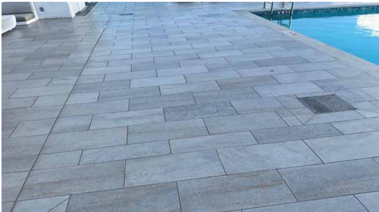
Pool Deck - Rooftop
