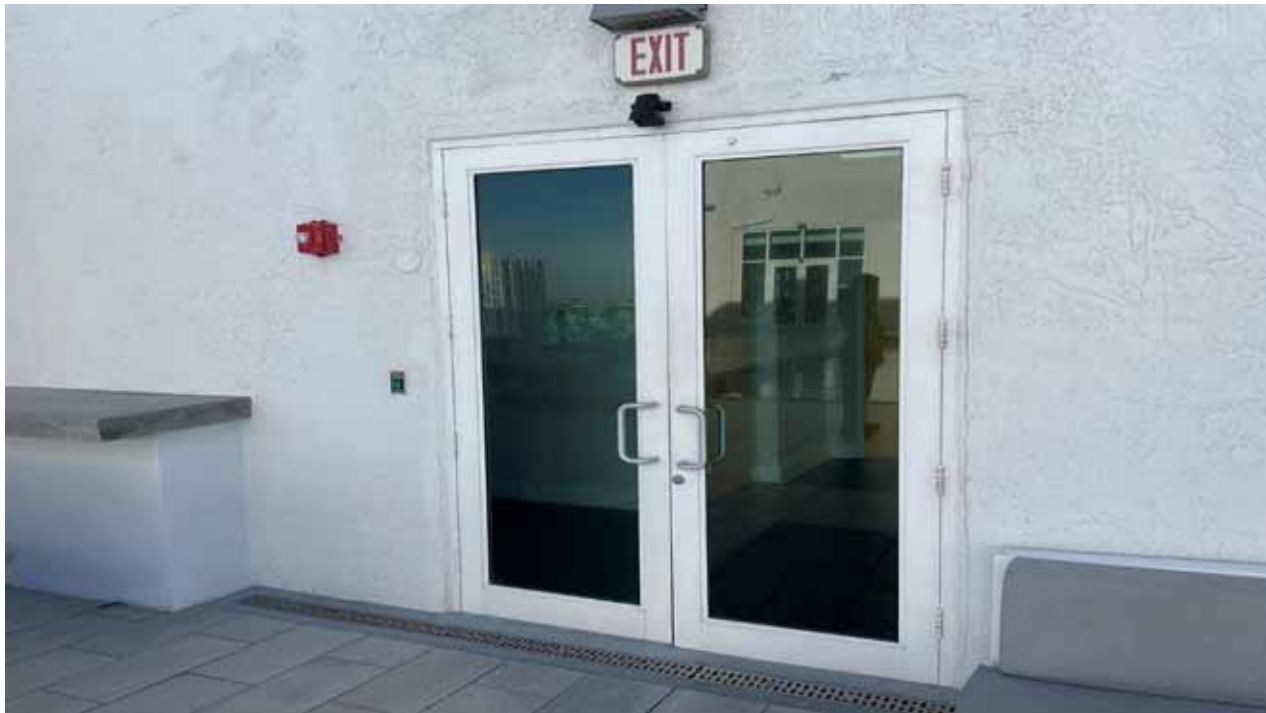
Doors - East Hallway
