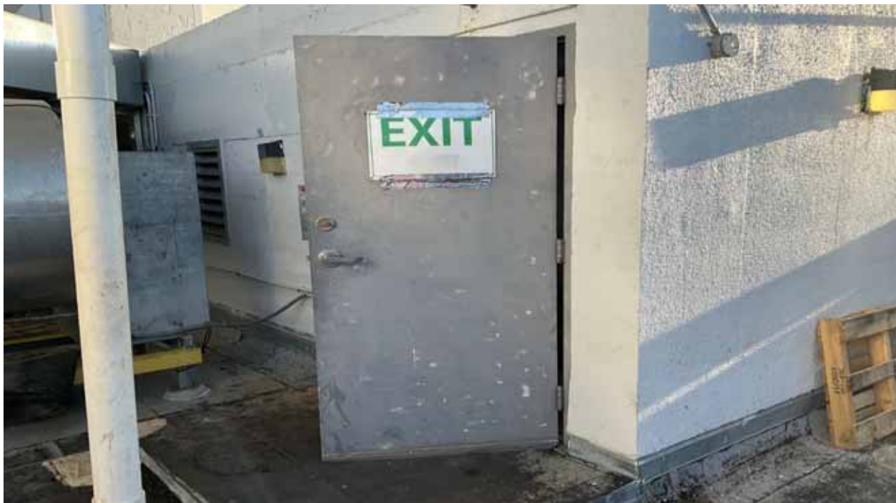
Door, Roof Access - West
