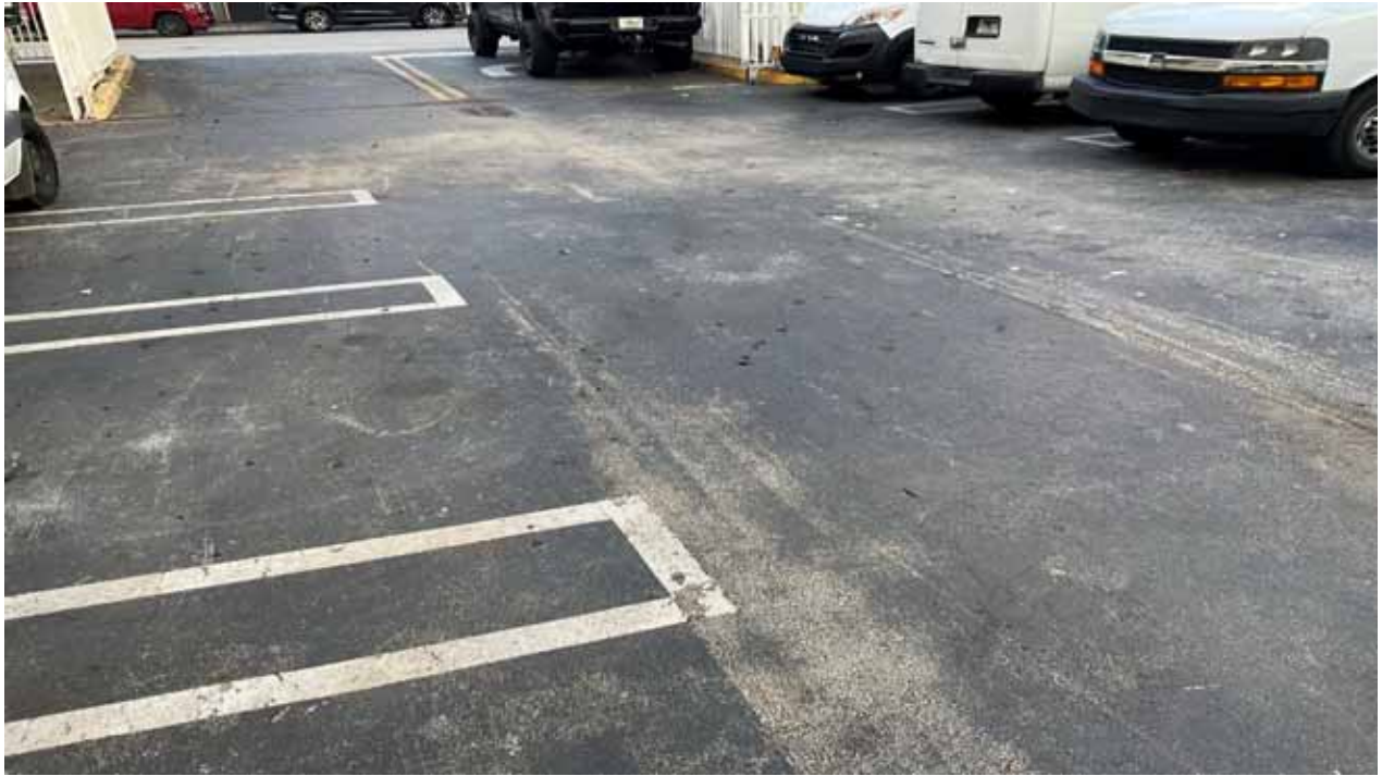
Pavement, Asphalt - Contractor Parking
