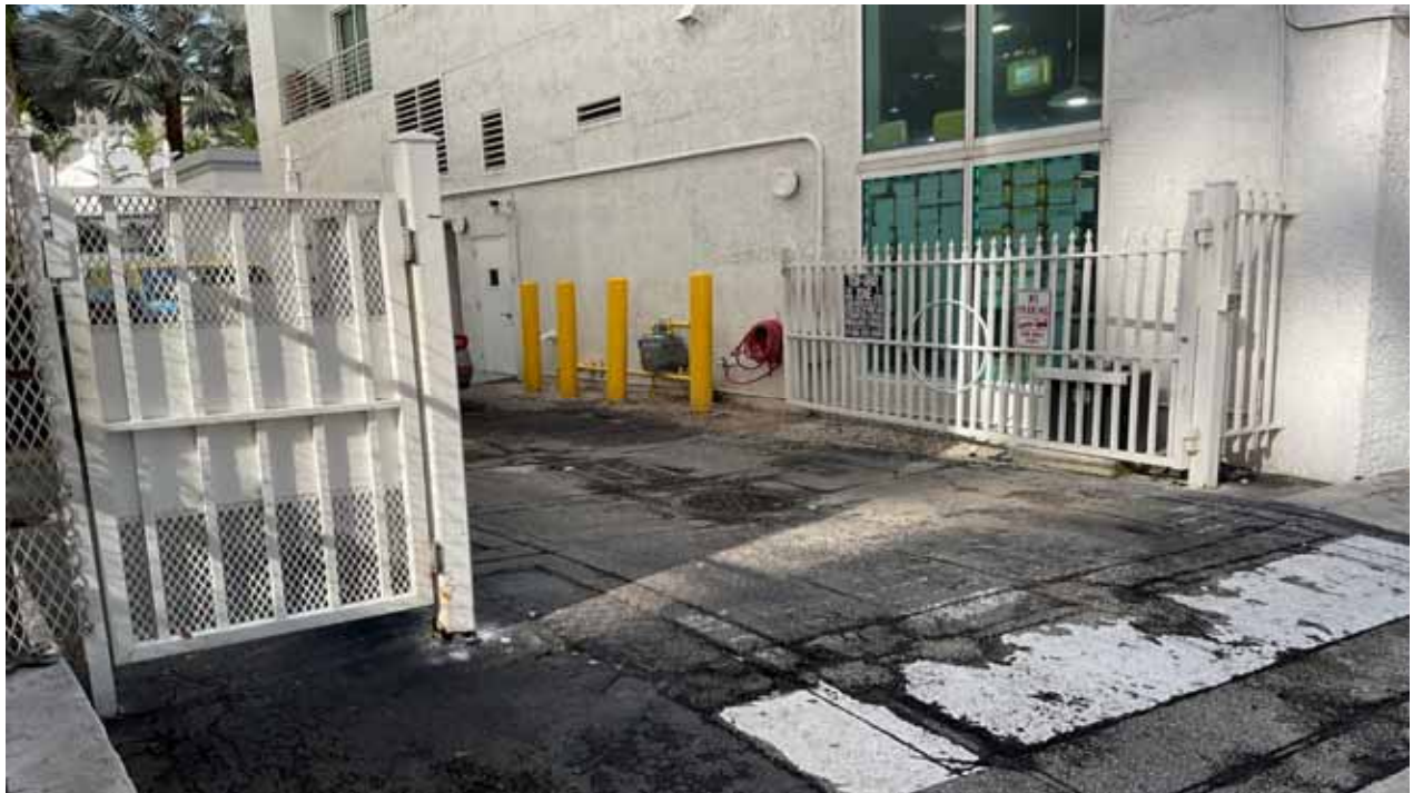
Fence & Gate - Receiving Area
