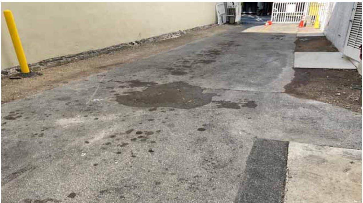
Pavement, Asphalt - Receiving Driveway
