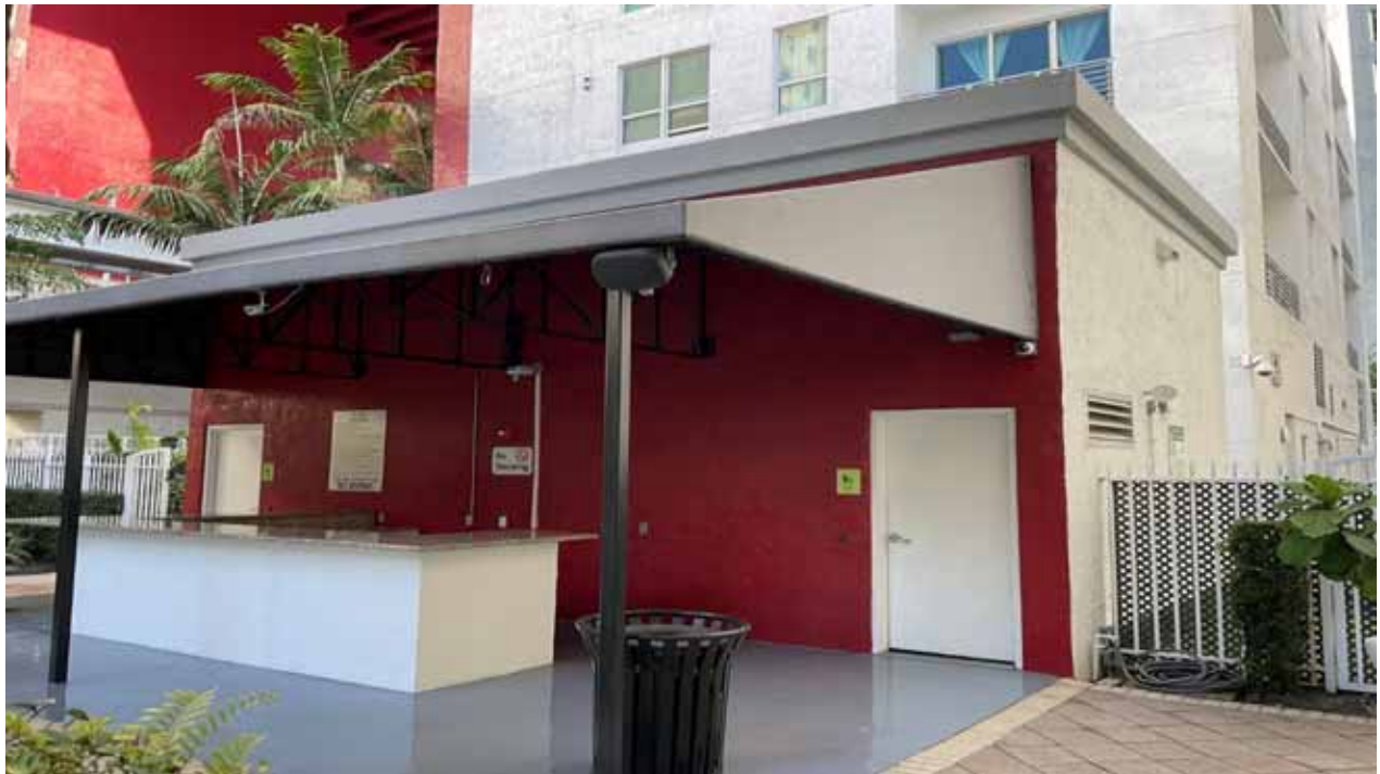
Pool Restroom Bldg - Ground Level
