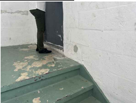
Reinforced Concrete Roof Deck
