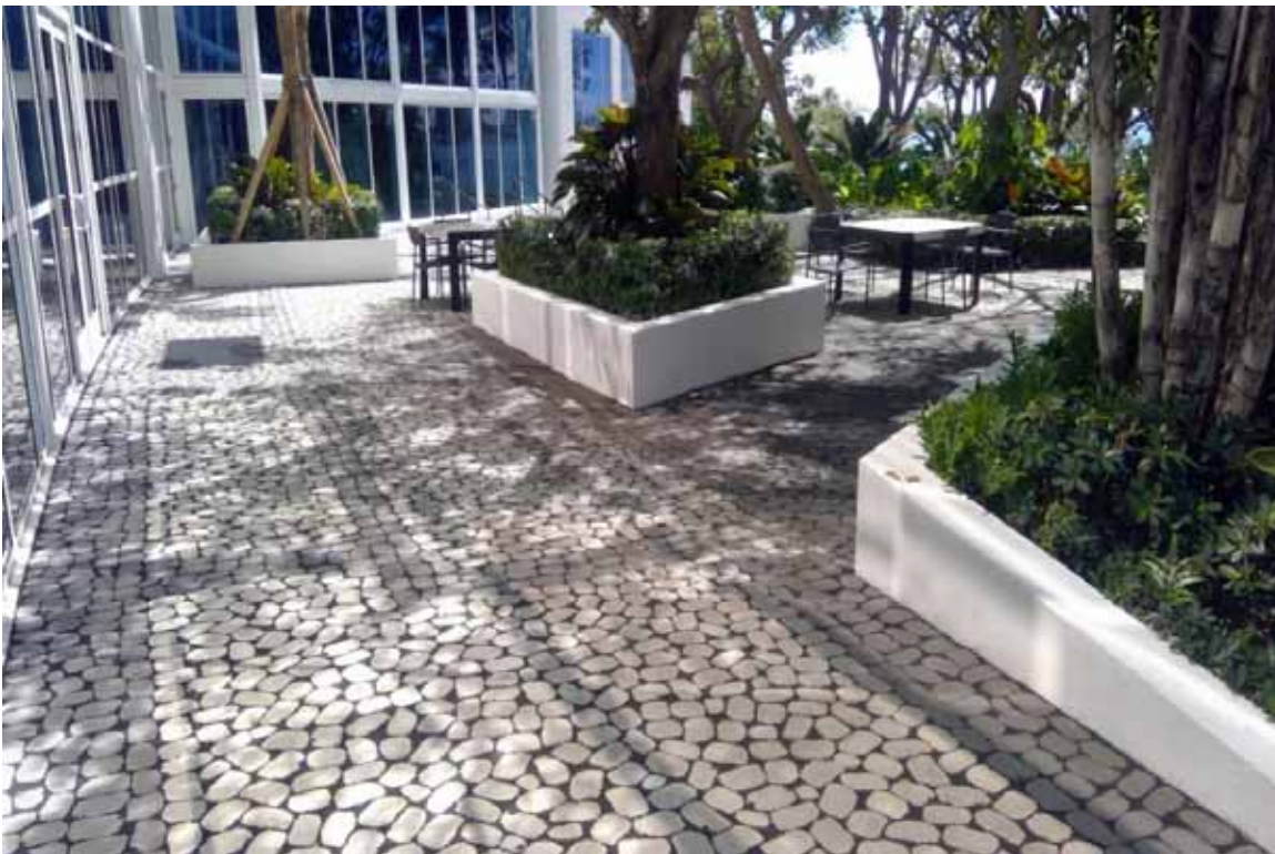
Pavers - Lobby Exterior
