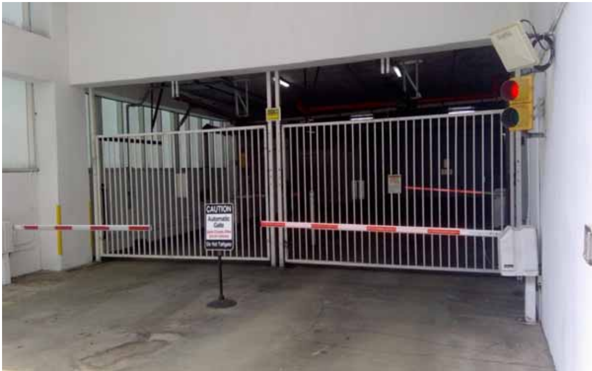
Gates - Garage Vehicular Access
