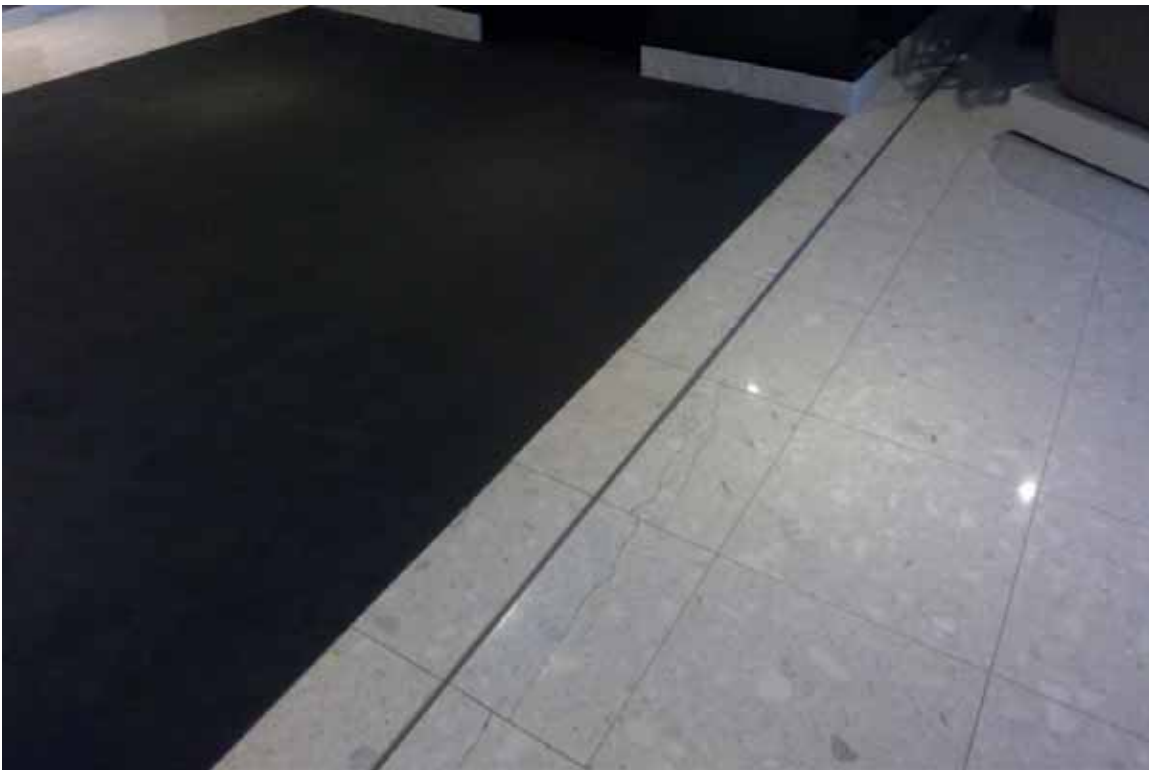
Expansion Joint - Mezzanine
