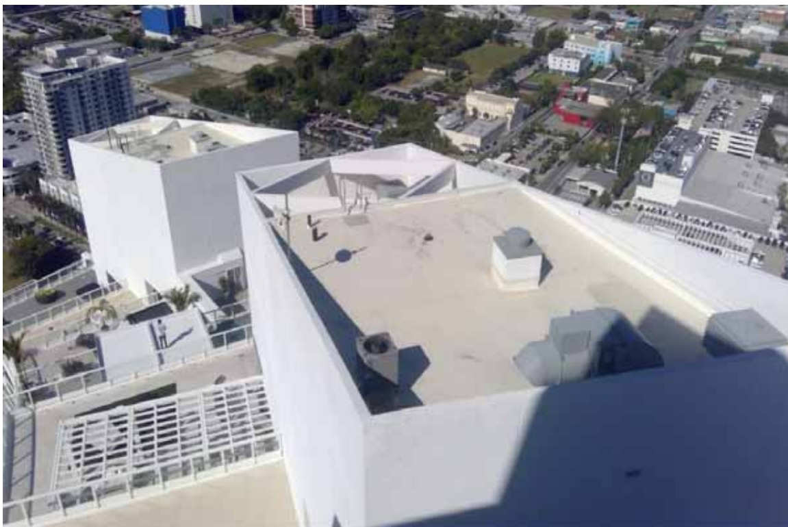
Roof - Center & South
