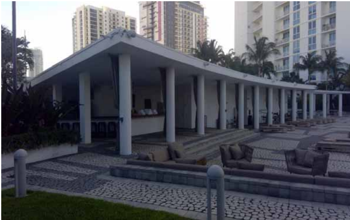
West Pool Restroom Bldg
