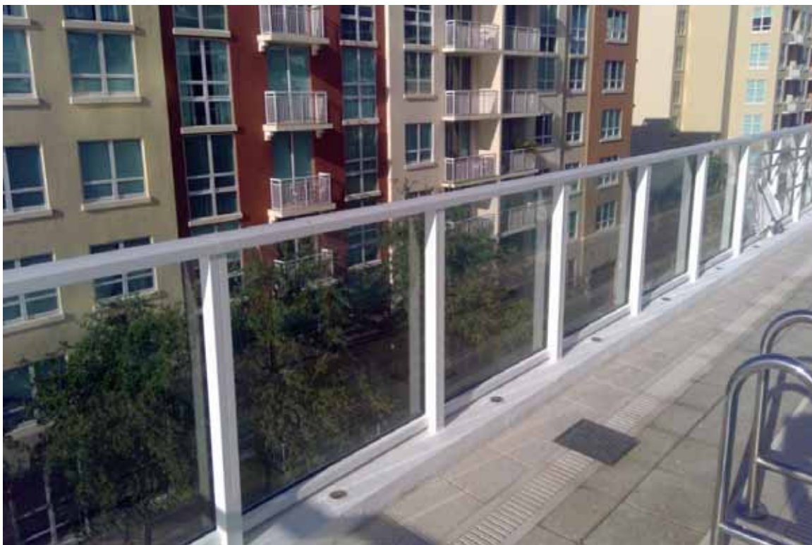
Railing - East Pool
