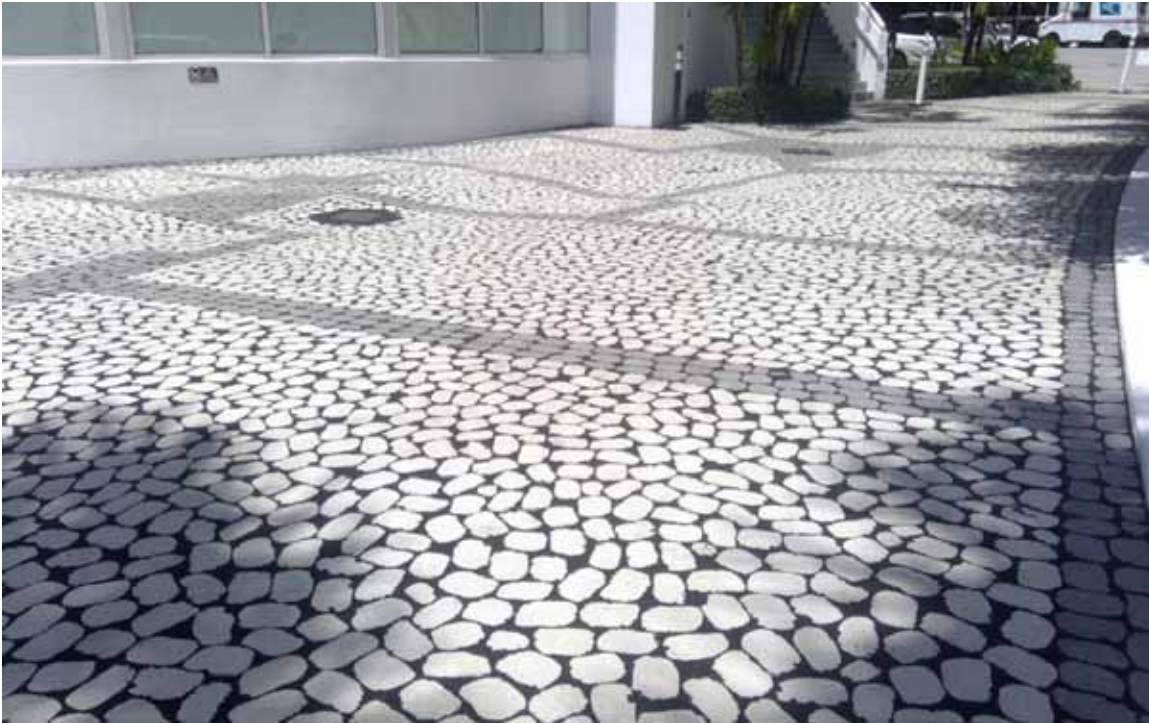
Pavers - Commercial Space B
