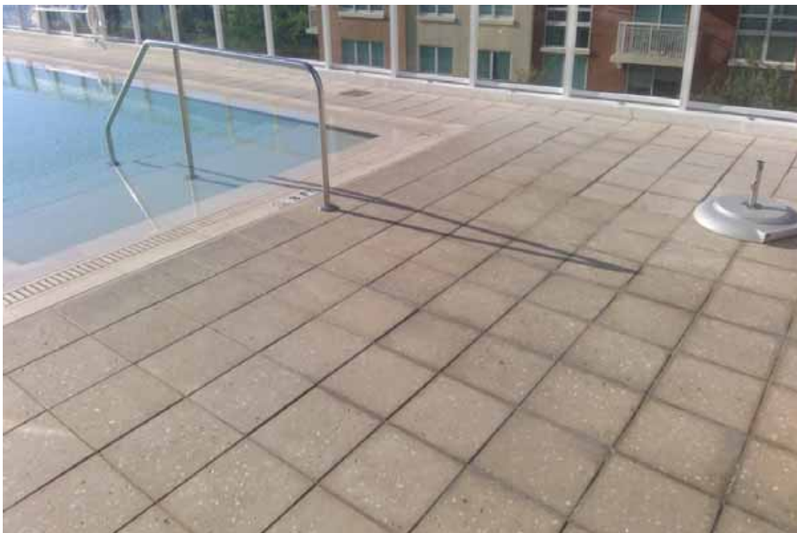
East Pool Deck
