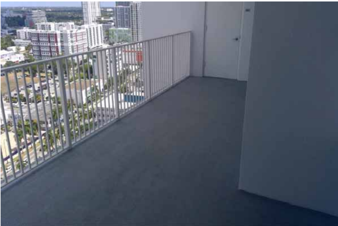
Walkway - Service, Upper Floor
