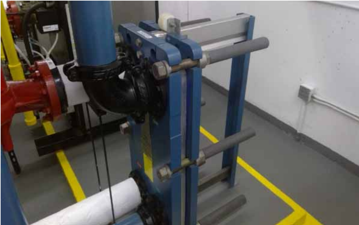
Heat Exchanger - Condensing Water
