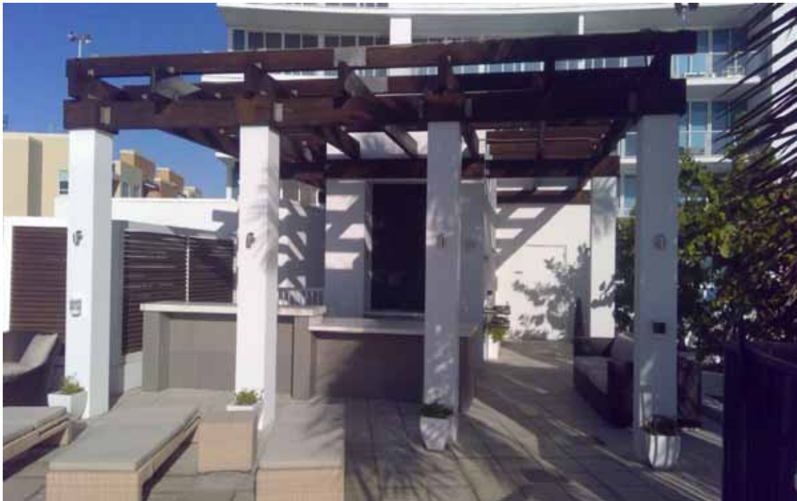
East Pool Restroom Bldg
