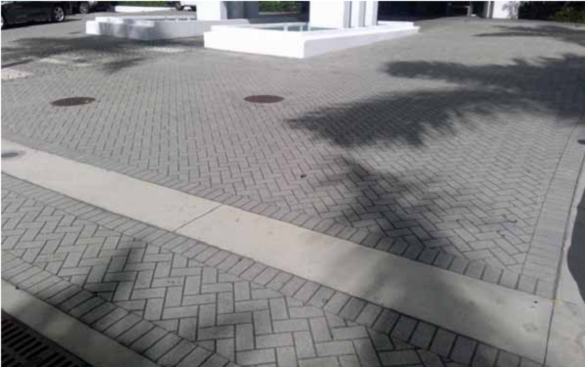
Pavers - Entry Plaza
