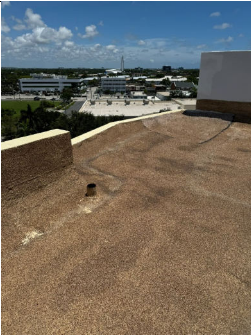
Image 16: Roof parapet detail.
