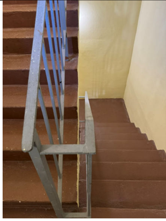
Image 15: Interior emergency stairs.
