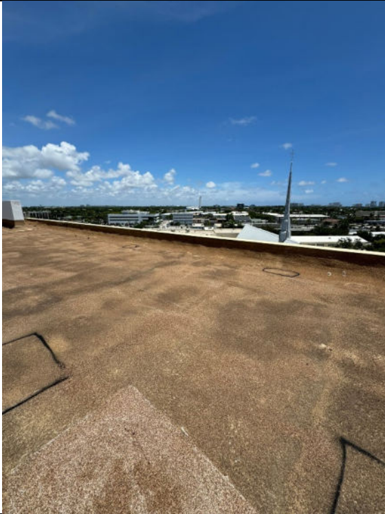
Image 18: General view of the roof.
