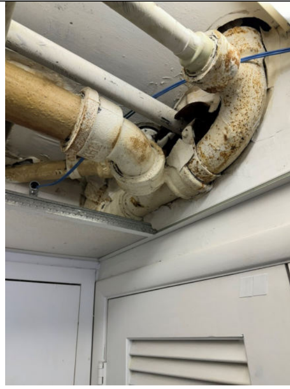
Image 7: Building sewer lines are cast iron.
