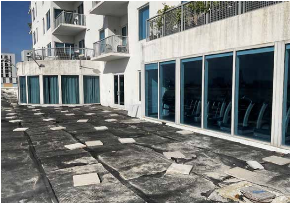
Windows & Doors - Fitness Center & Club Room
