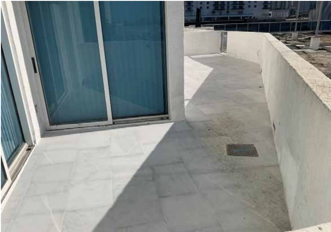
Unit Balcony - 6th Floor
