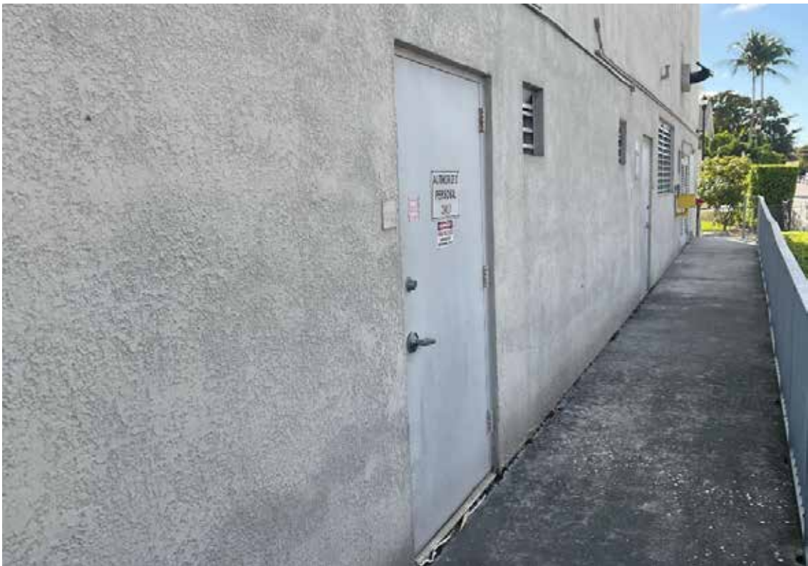
Door - Main Electrical Room
