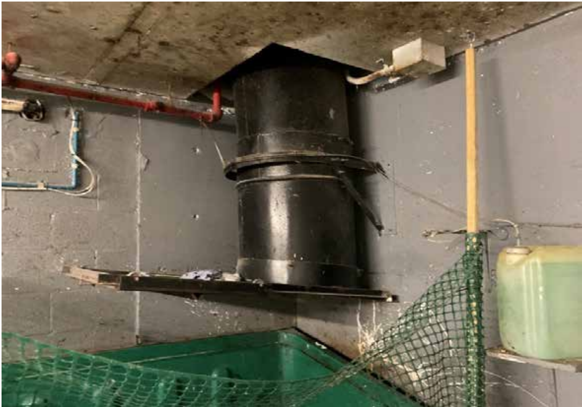
Trash Chute Guillotine
