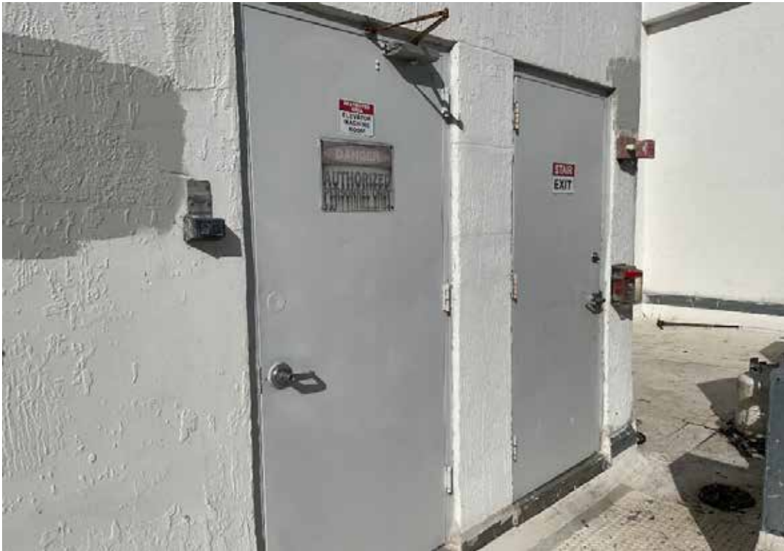
Doors - Elevator Equipment & Roof Access
