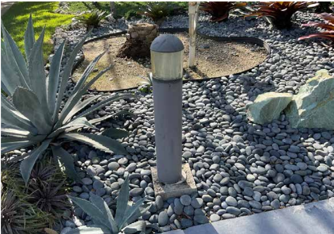
Light Bollard - Walkway
