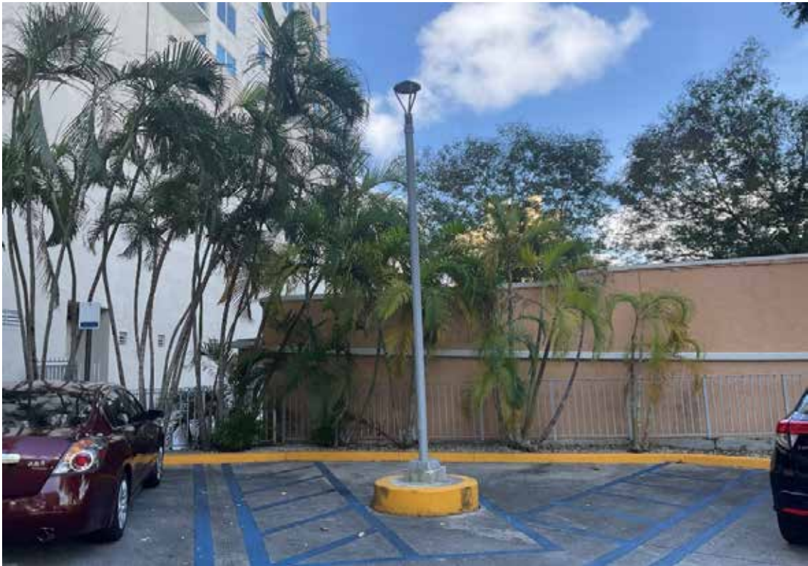
Light Pole & Fixture - Driveway
