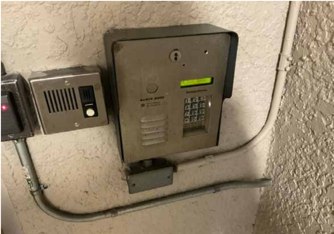
Access Control - Enterphone, FOB Reader & Intercom
