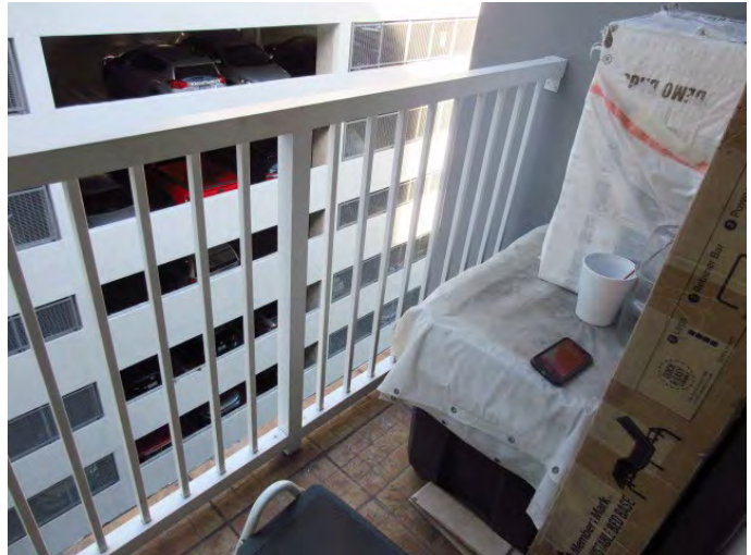
GENERAL VIEW OF BALCONY RAILING
