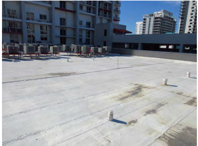
GENERAL VIEW OF BUILDING EXTERIOR FINISHES
