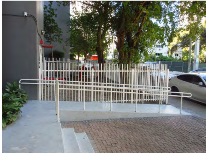
GENERAL VIEW OF SITE FENCE AND RAMP RAILING
