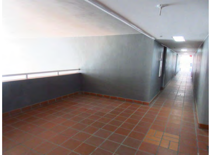
VIEW OF ELEVATED WALKWAY
