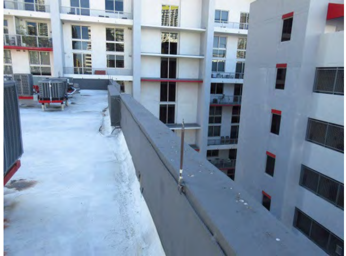
GENERAL VIEW OF ROOF PARAPET WALL
