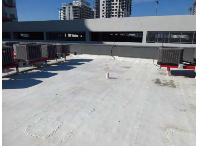
GENERAL VIEW OF ROOF COVERING
