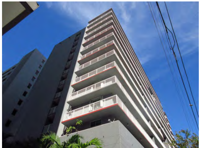
VIEW OF BUILDING EXTERIOR FINISHES
