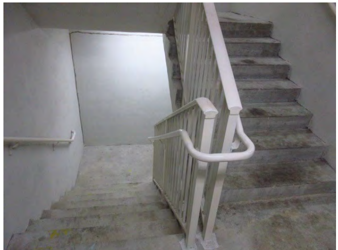
VIEW OF STAIRS
