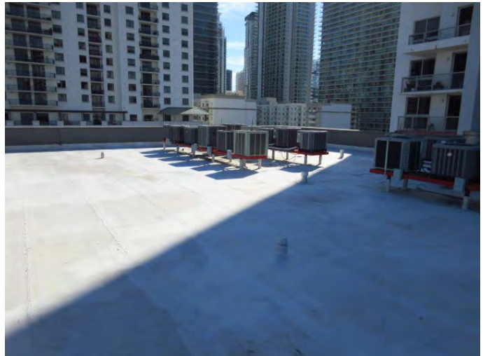
VIEW OF ROOF COVERING
