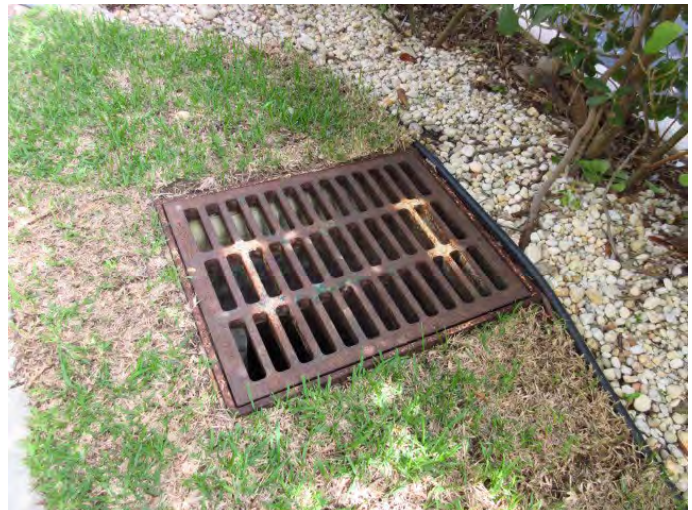
GENERAL VIEW OF STORM WATER INLET
