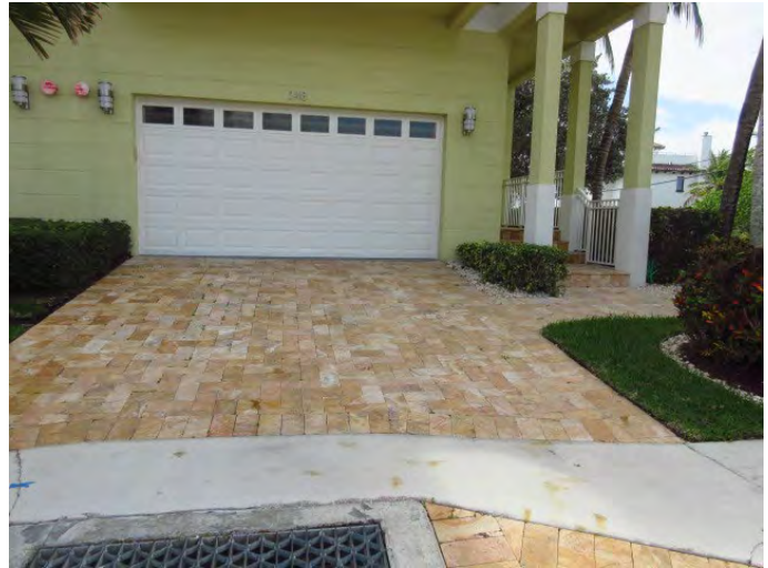
GENERAL VIEW OF TYPICAL UNIT DRIVEWAY
