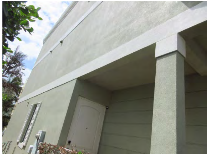
VIEW OF BUILDING EXTERIOR FINISHES
