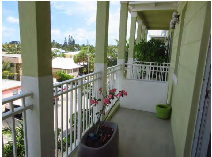
GENERAL VIEW OF TYPICAL BALCONY
