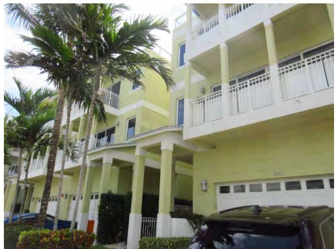
VIEW OF BUILDING EXTERIOR FINISHES
