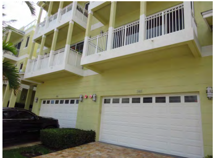
GENERAL VIEW OF TYPICAL UNIT GARAGES
