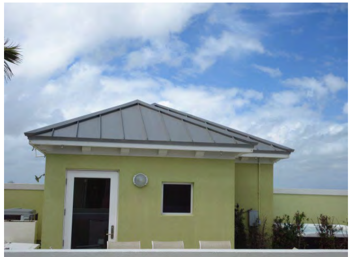
VIEW OF PITCHED ROOF COVERING
