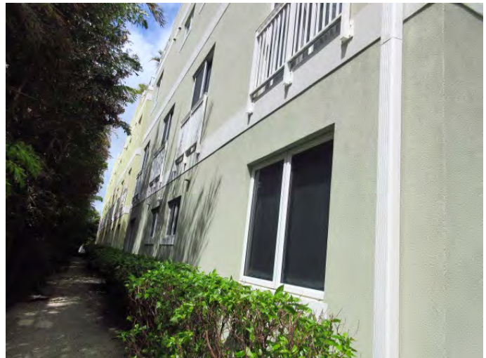
VIEW OF BUILDING EXTERIOR FINISHES
