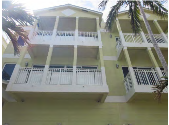
GENERAL VIEW OF BUILDING EXTERIOR FINISHES
