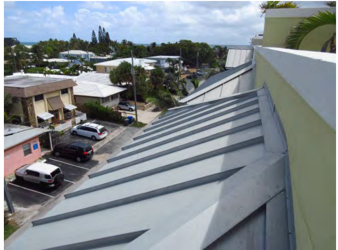
VIEW OF PITCHED ROOF COVERING
