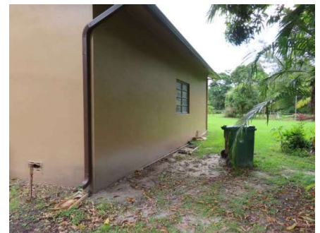
Rear Elevation Detached Garage
