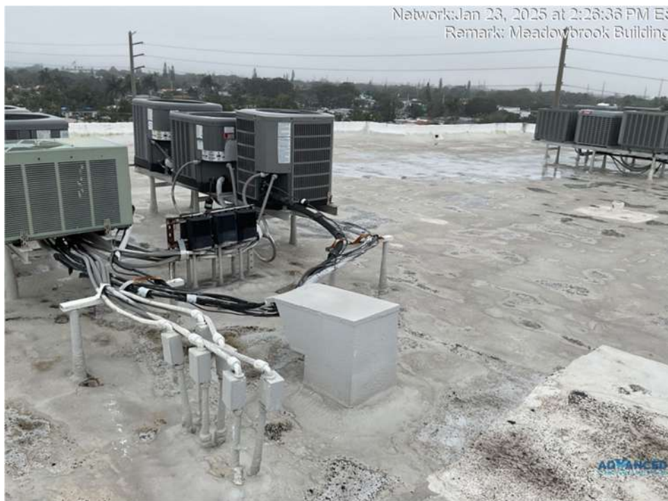
Figure 4. Roof and scooper in Good Conditions.
