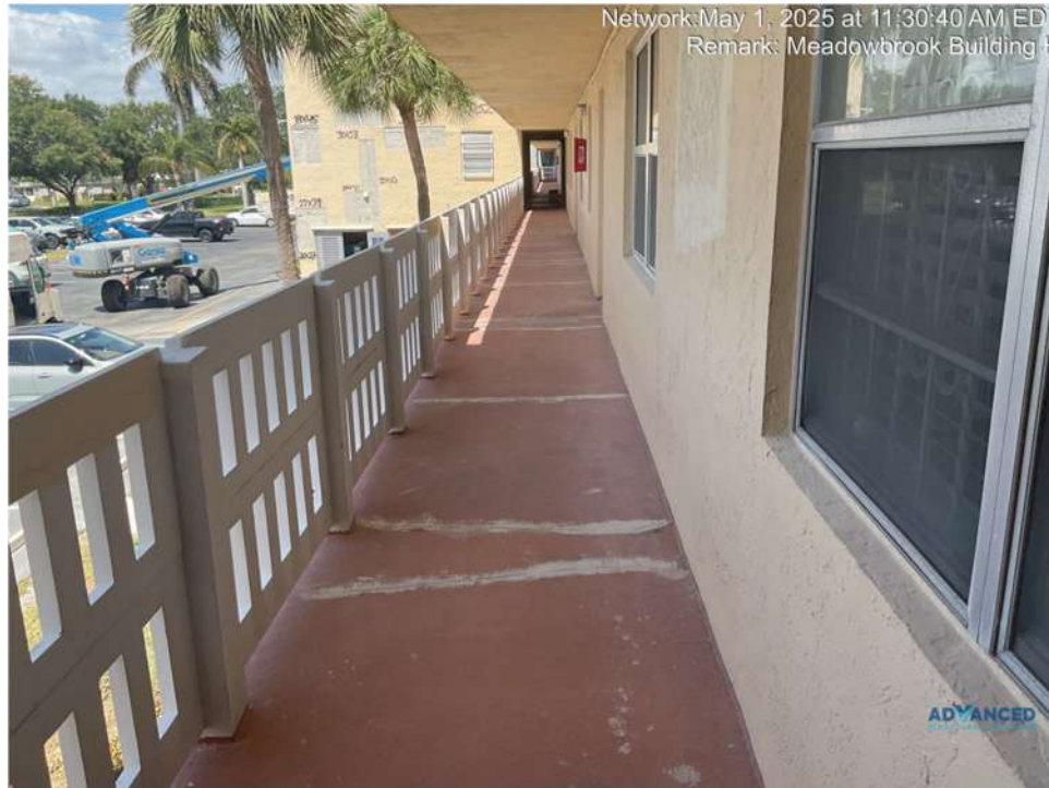
Figure 3. Walkways in Good Conditions.
