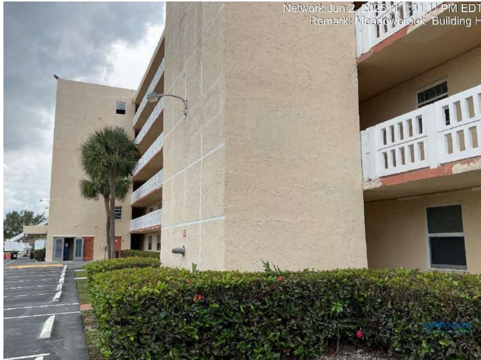
Figure 1. Building Overall Conditions - Good.
