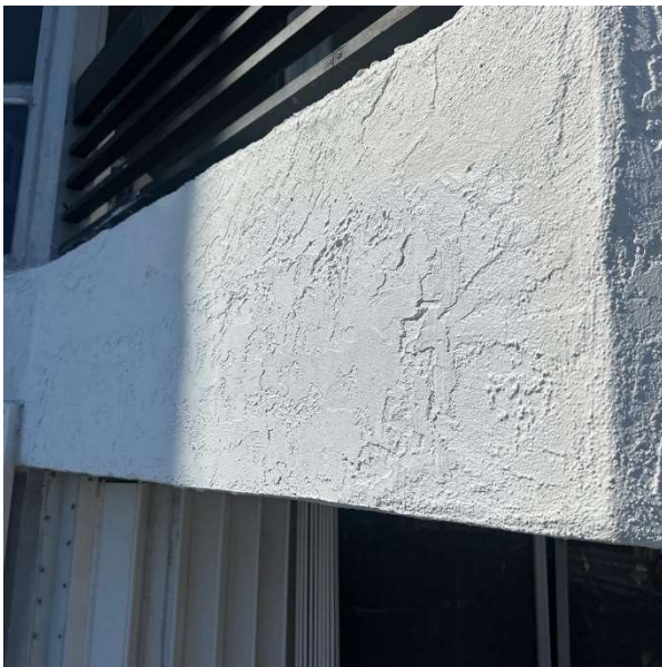
11. Edge of Slab and Knee Wall Repair
