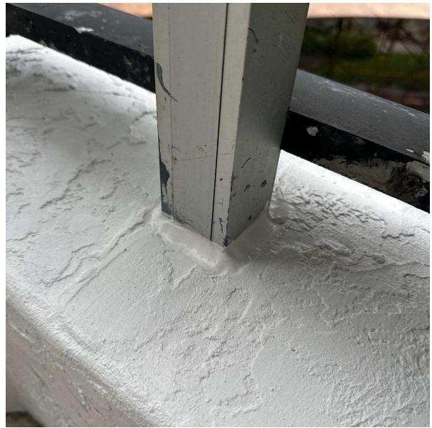
2. Post Pocket Repair
