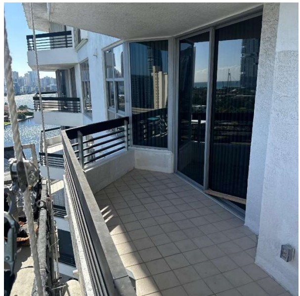
12. Overview of Repairs
