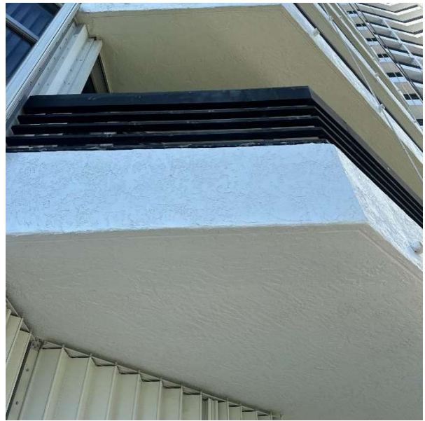
10. Edge of Slab and Knee Wall Repair
