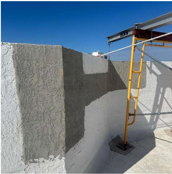
9. Parapet Wall Repair
