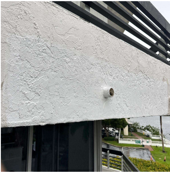
1. Concrete and Stucco Repair
