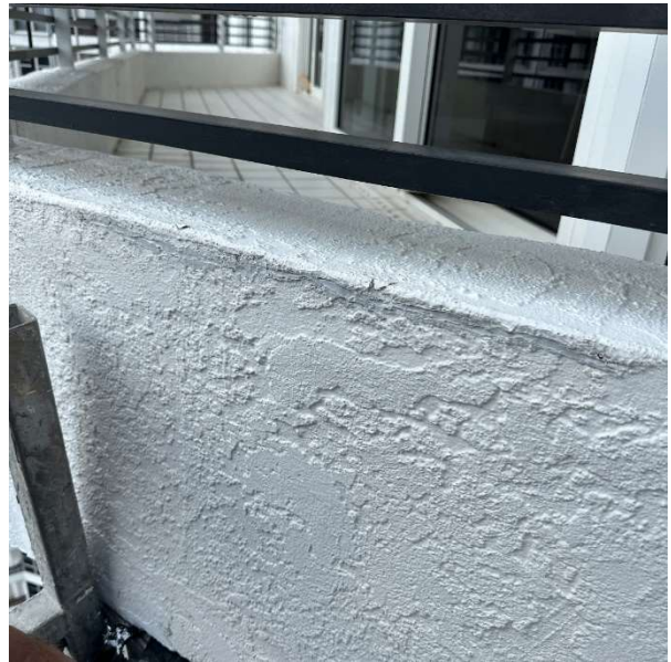
14. Crack Repair
