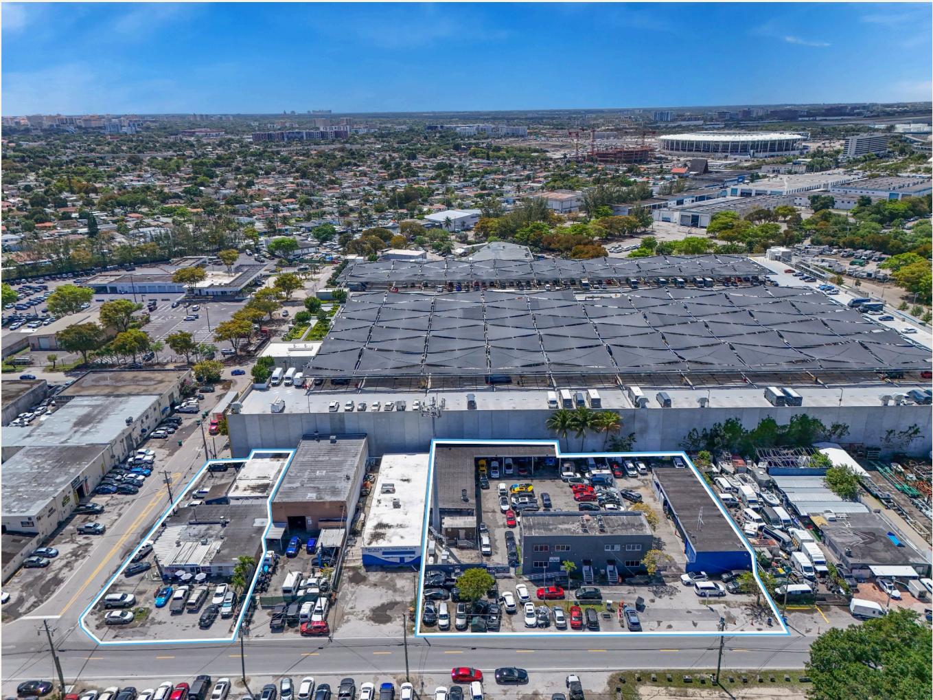
Combined aerial of the Miami River Strategic Acquisition — 3326 NW South River Drive (right parcel) and its adjoining lot (left parcel), both outlined in blue, fronting NW South River Drive.
