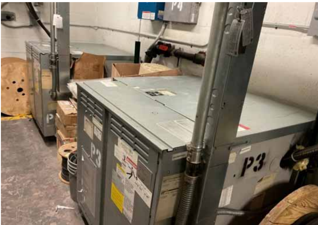
Elevator Equip - Passenger 3-4
