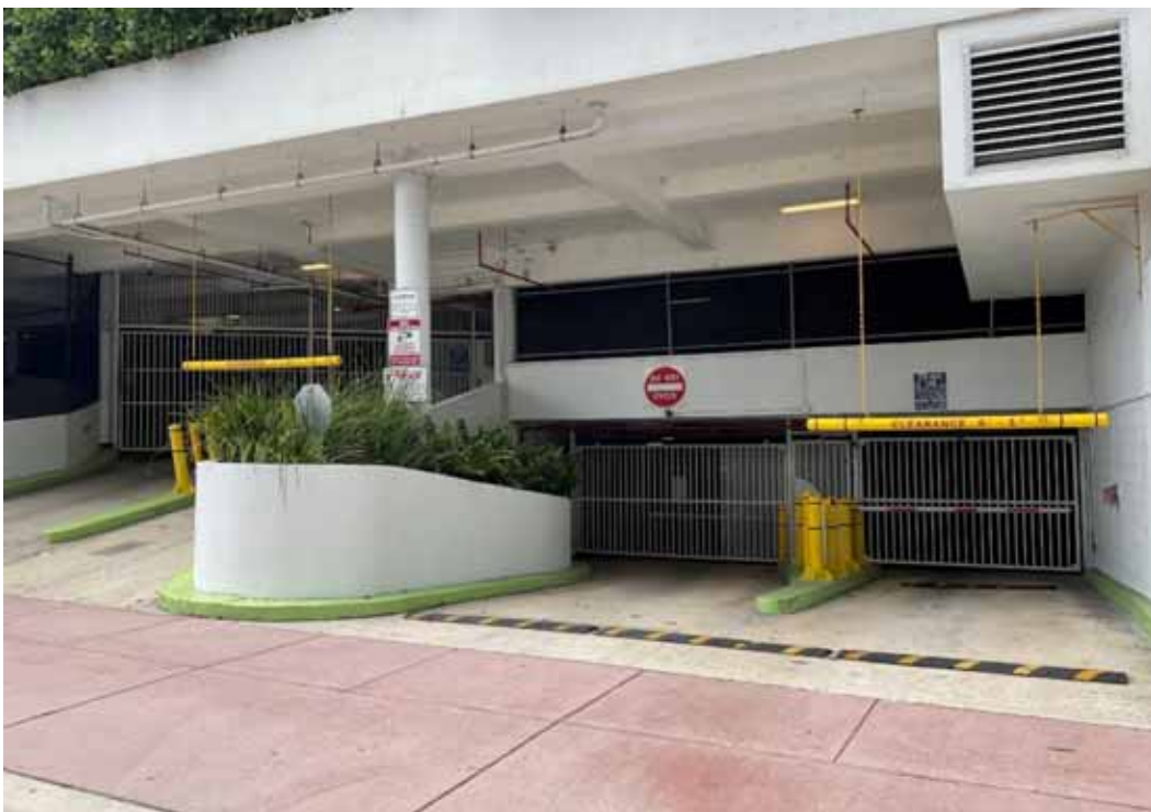
Garage Entry - North
