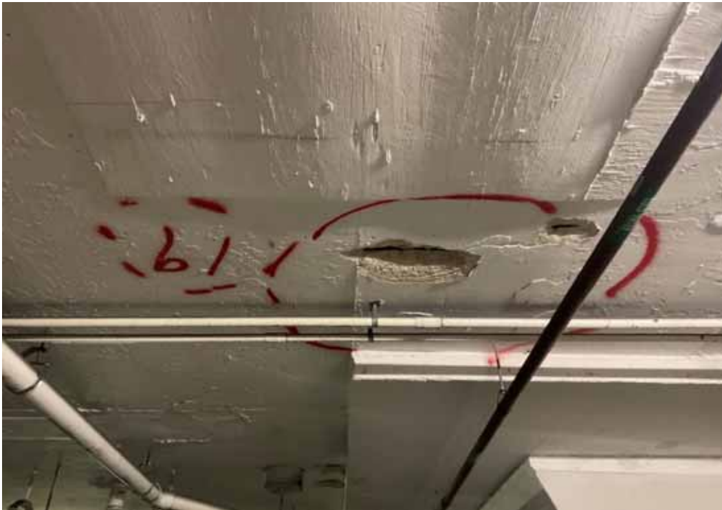
Spalling Concrete
