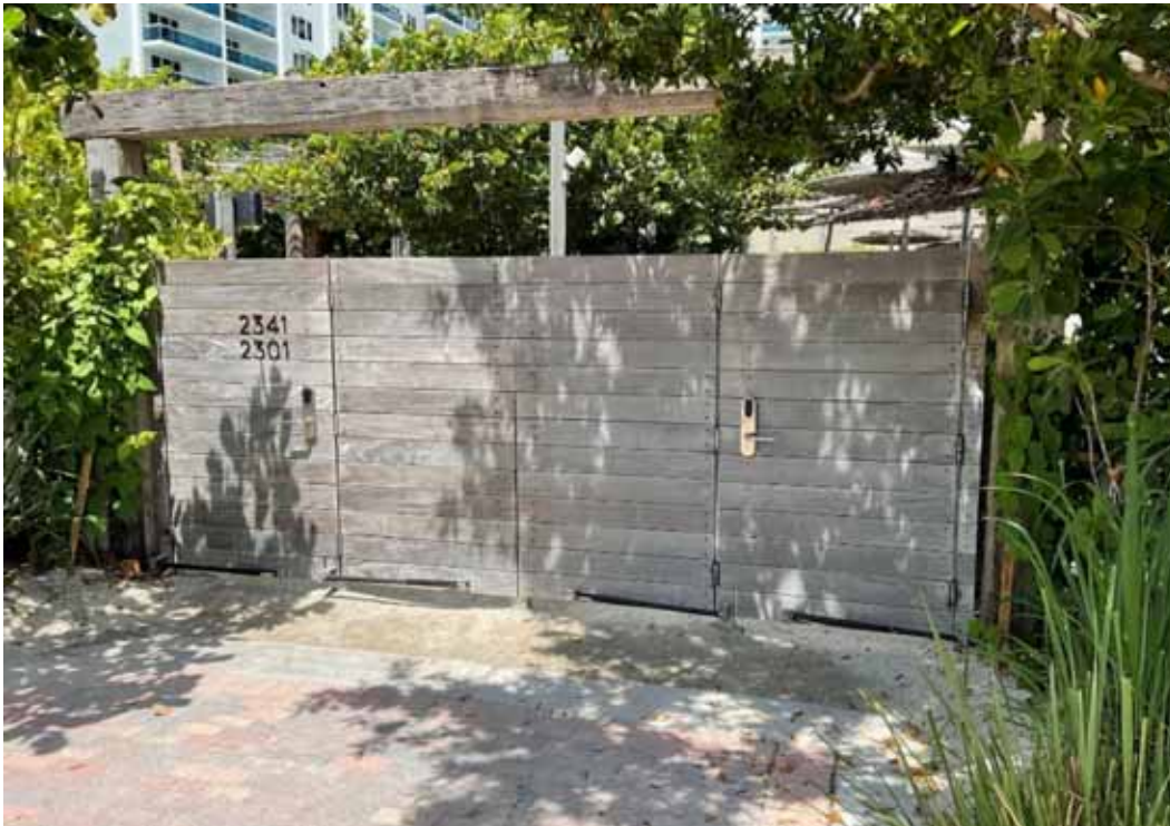
Gate - Beach Access
