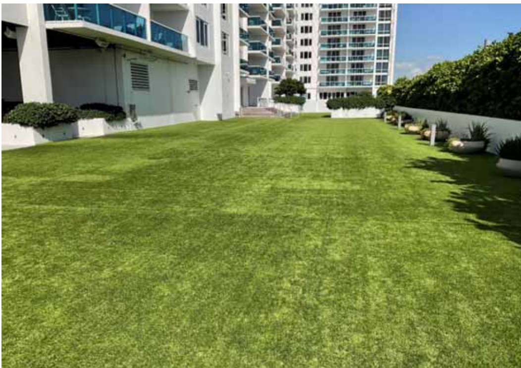
North Terrace Deck
