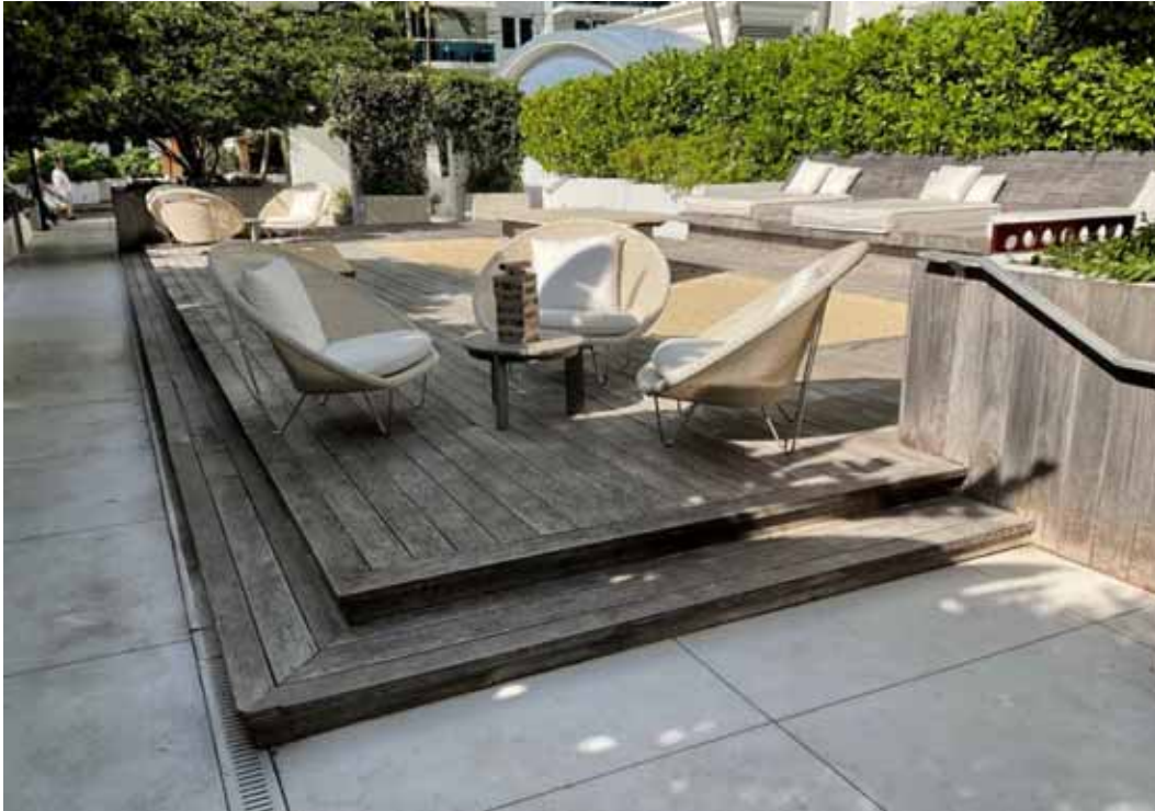
Main Pool Elevated Decking
