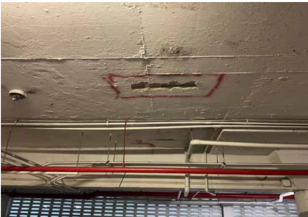
Spalling Concrete
