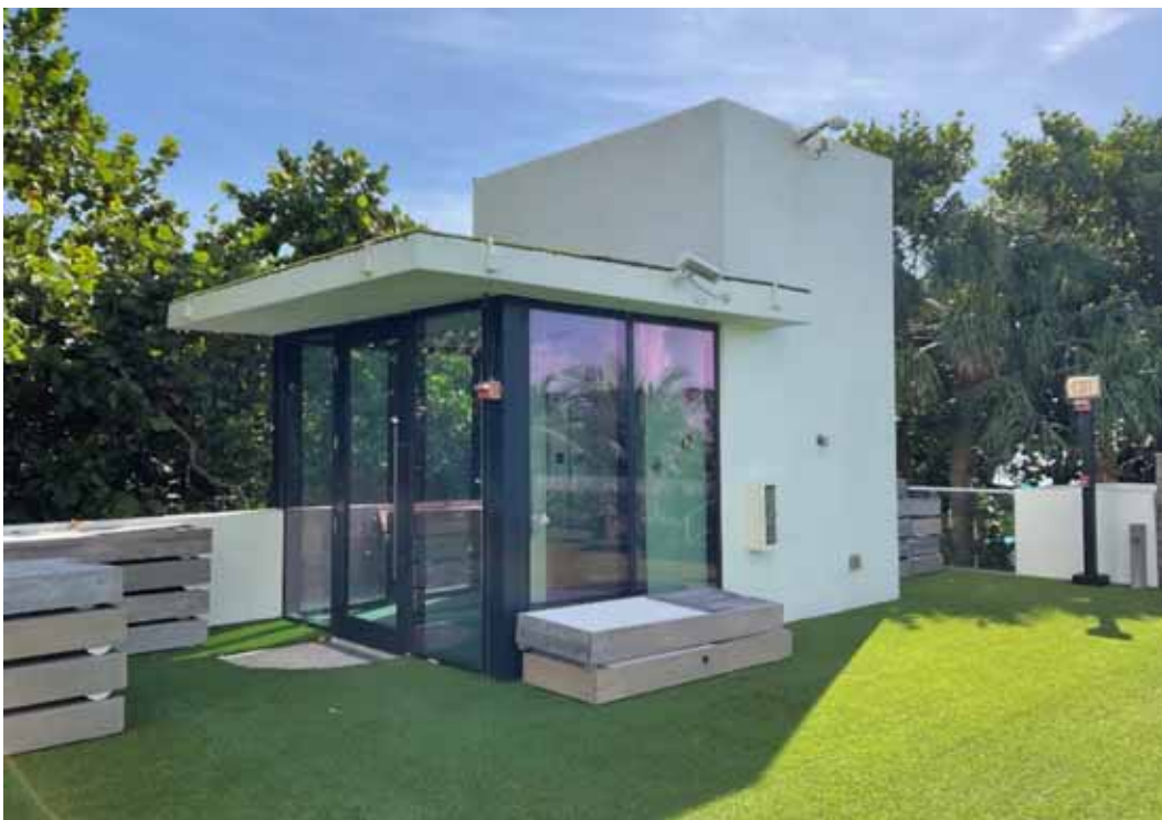
North Terrace Elevator
