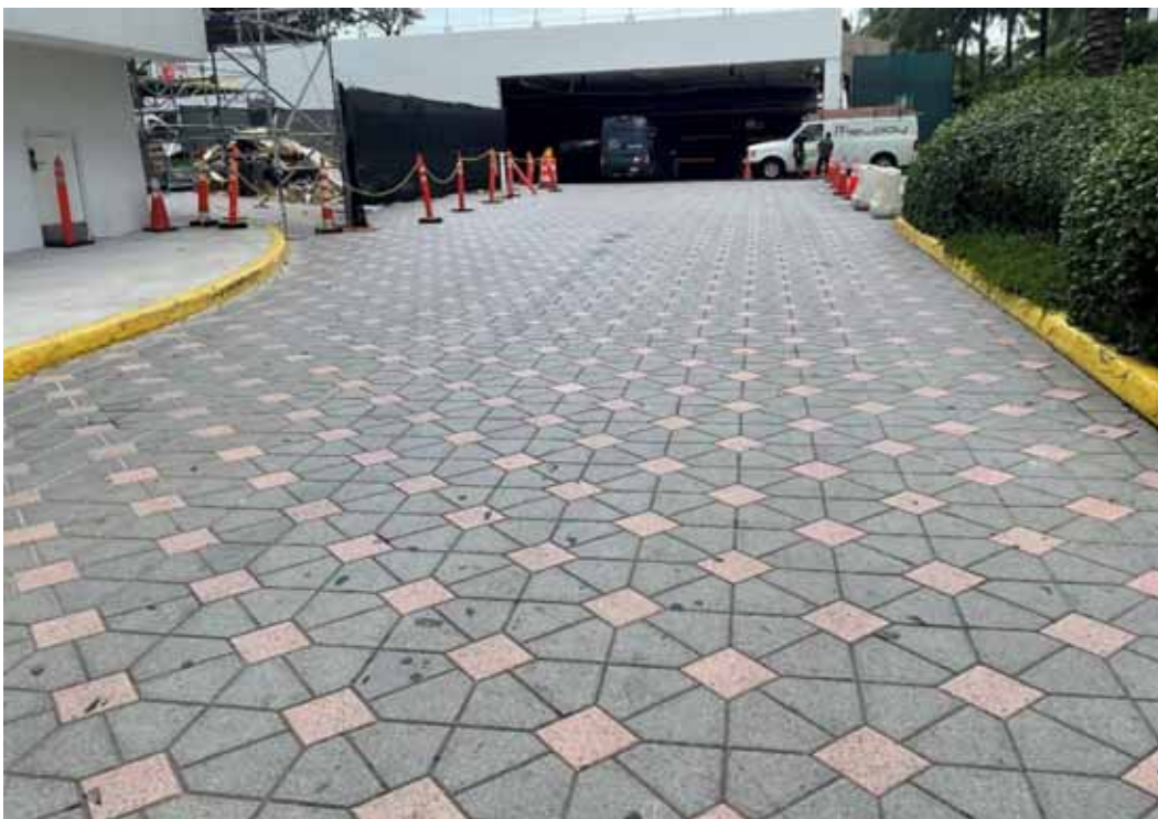
Pavers - South Entry
