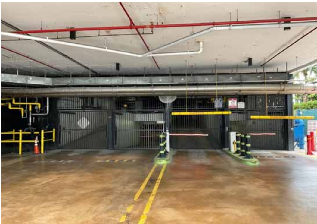
Garage Entry - South
